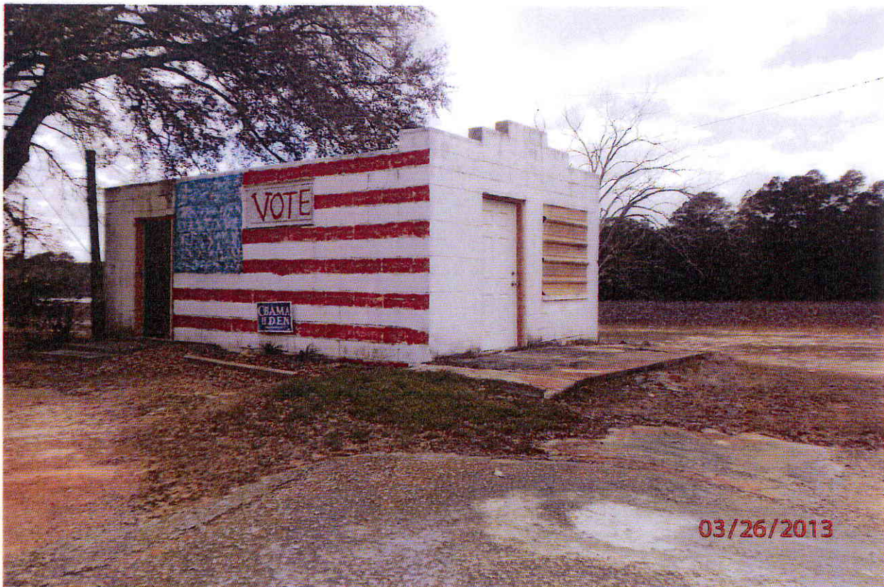
Figure 2: Side of the Subject Site.
