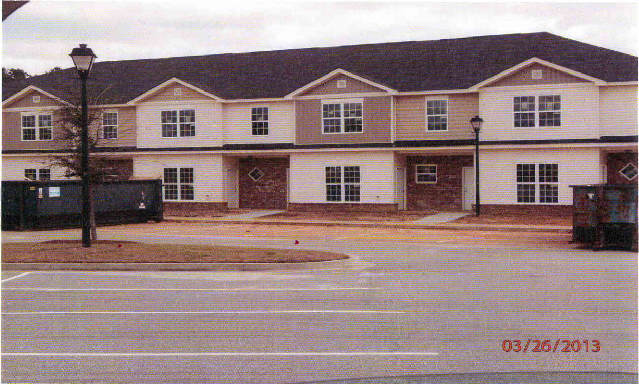
Figure 3: Building under construction.
