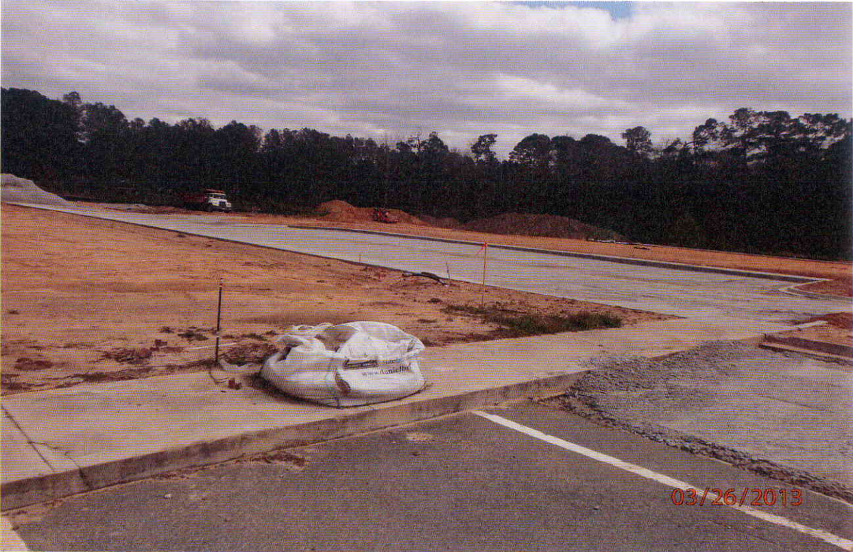
Figure 4: Construction site at rear of subject property for future buildings.
