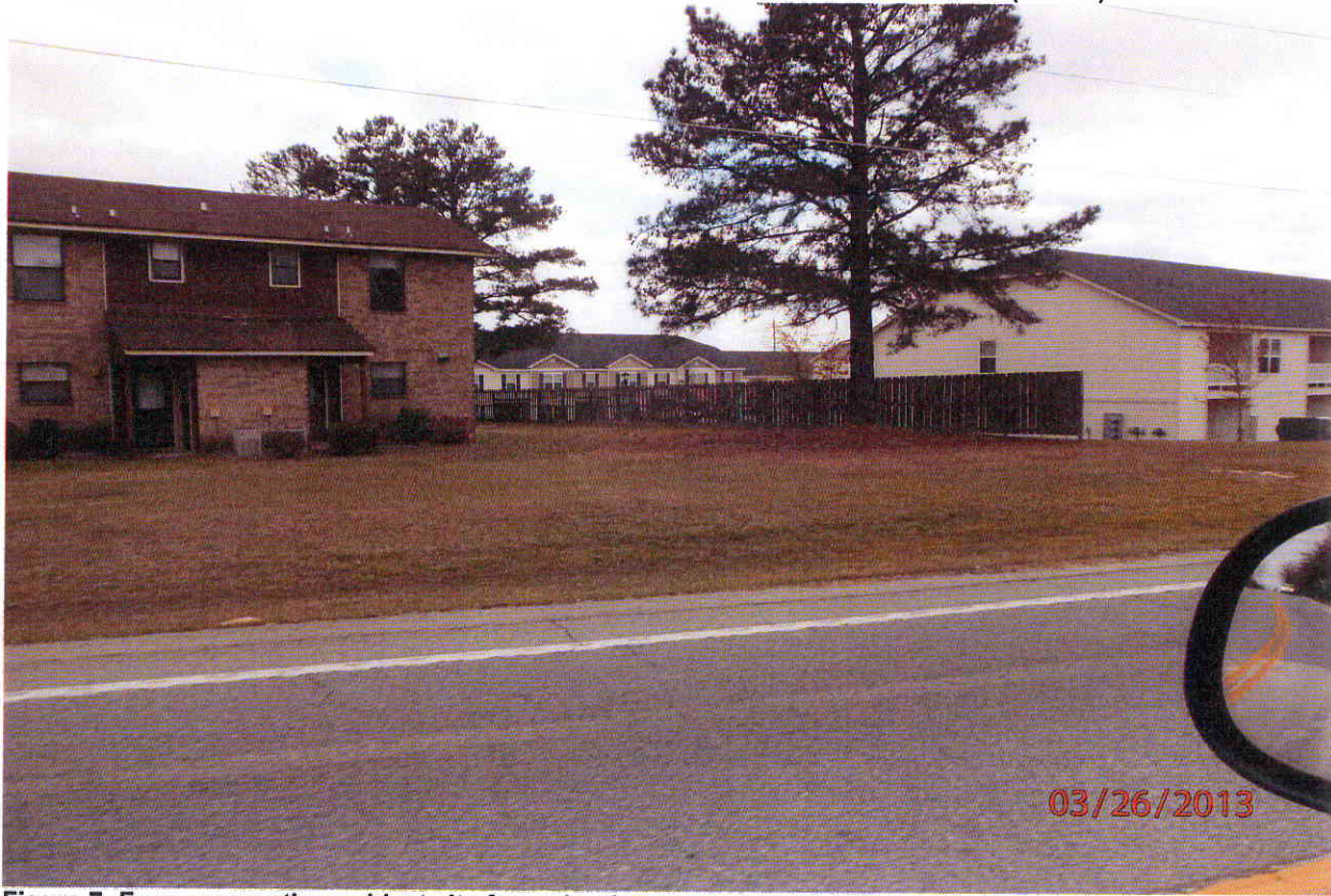
Figure 7: Fence separating subject site from abutting apartment complex.
