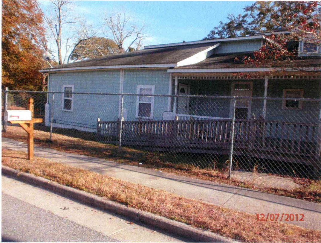
Figure 4: East Side of Building.
