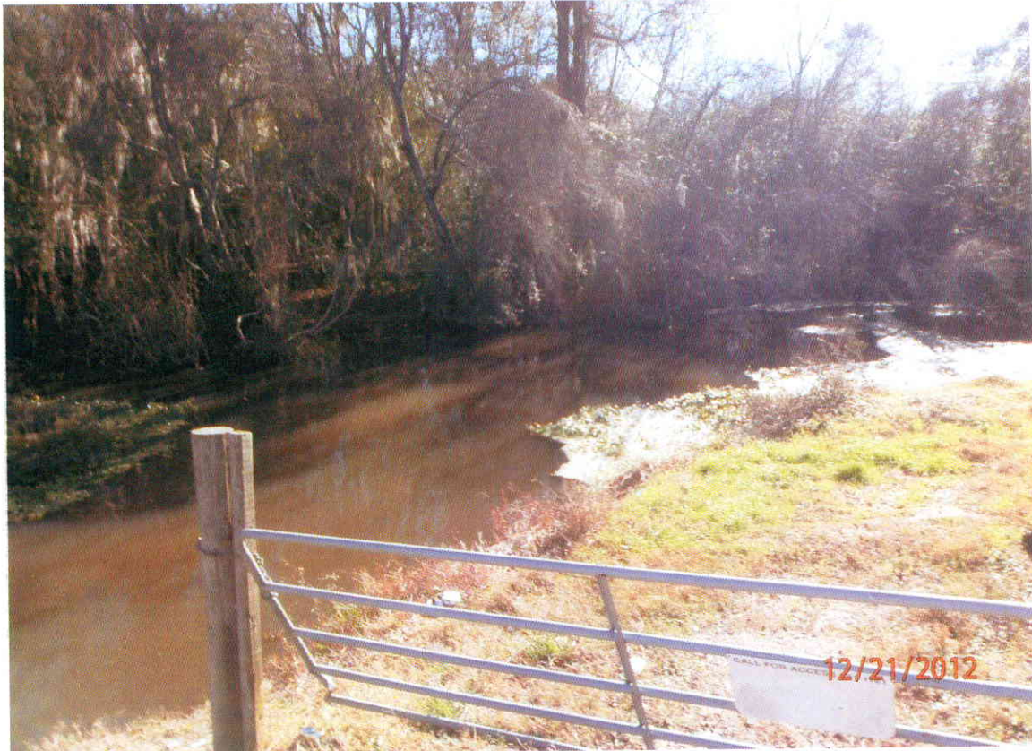
Figure 4: Storm Water Basin.
