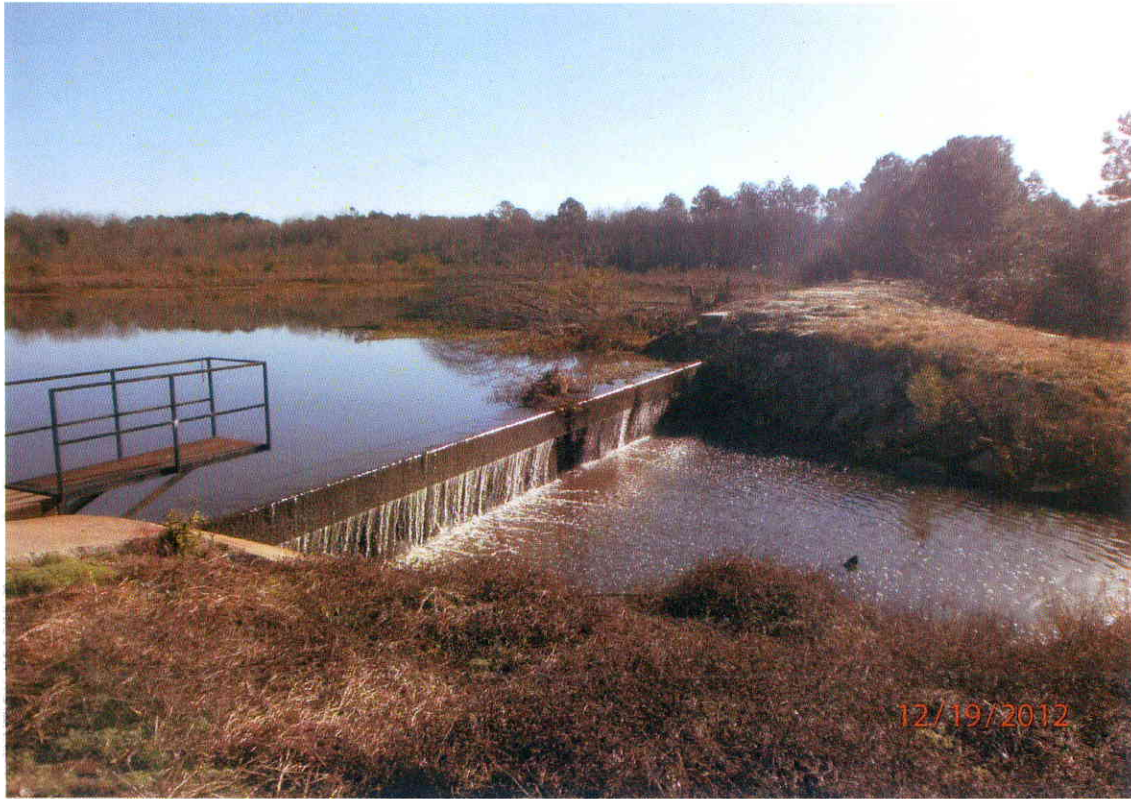
Figure 4: Storm Water Detention.
