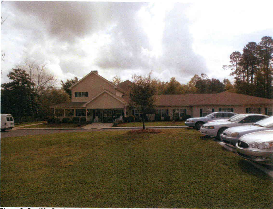
Figure 2: Gentilly Gardens (Rear Portion to be combined with Subject Site.)
