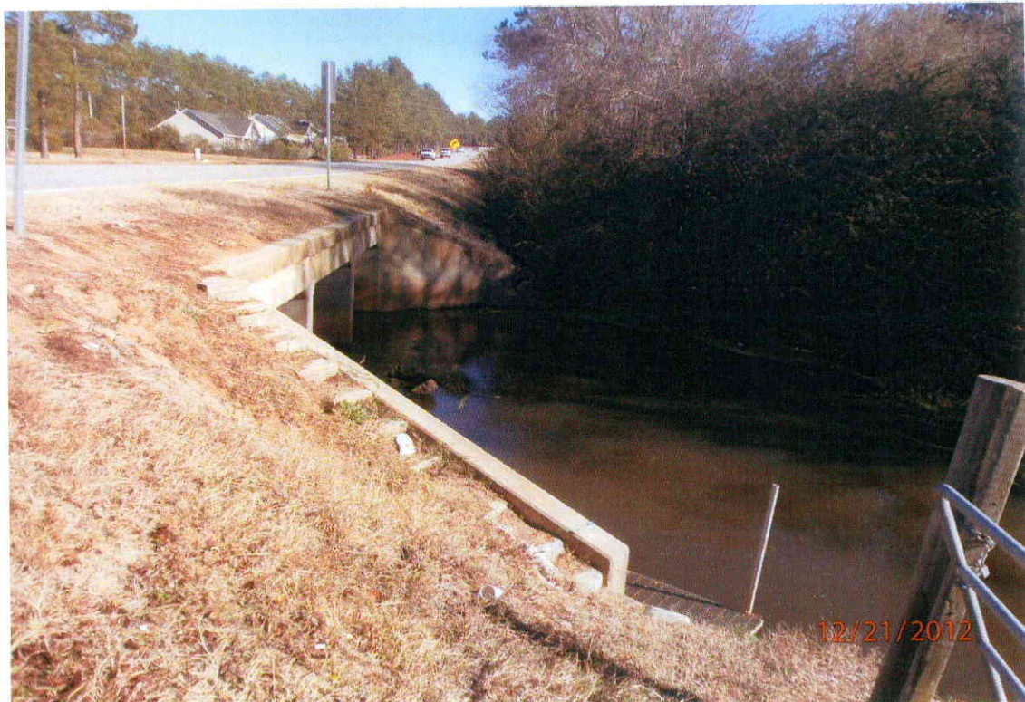
Figure 3: Water Crossing under Langston Chapel from Birds Pond.
