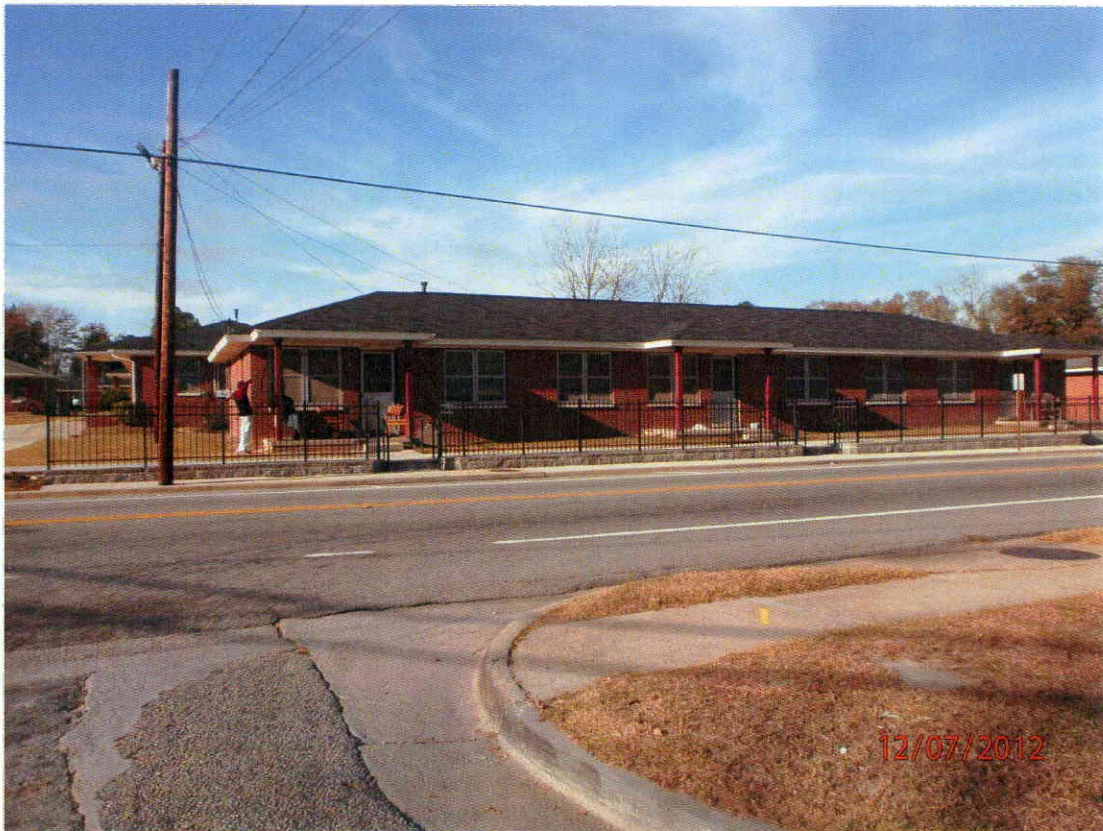
Figure 4: Statesboro Housing Authority across Johnson Street North of the Subject Site.
