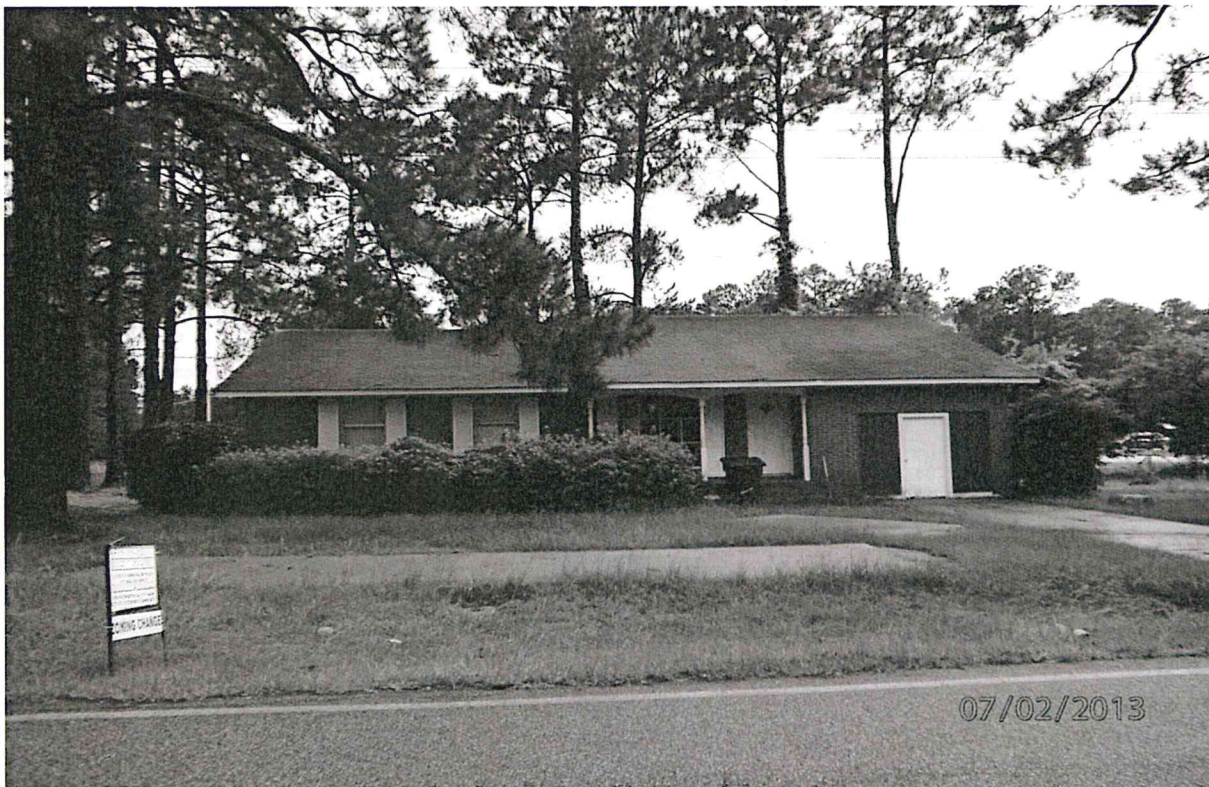
Figure 2: Single Family Home located on Property – Catherine Avenue.
