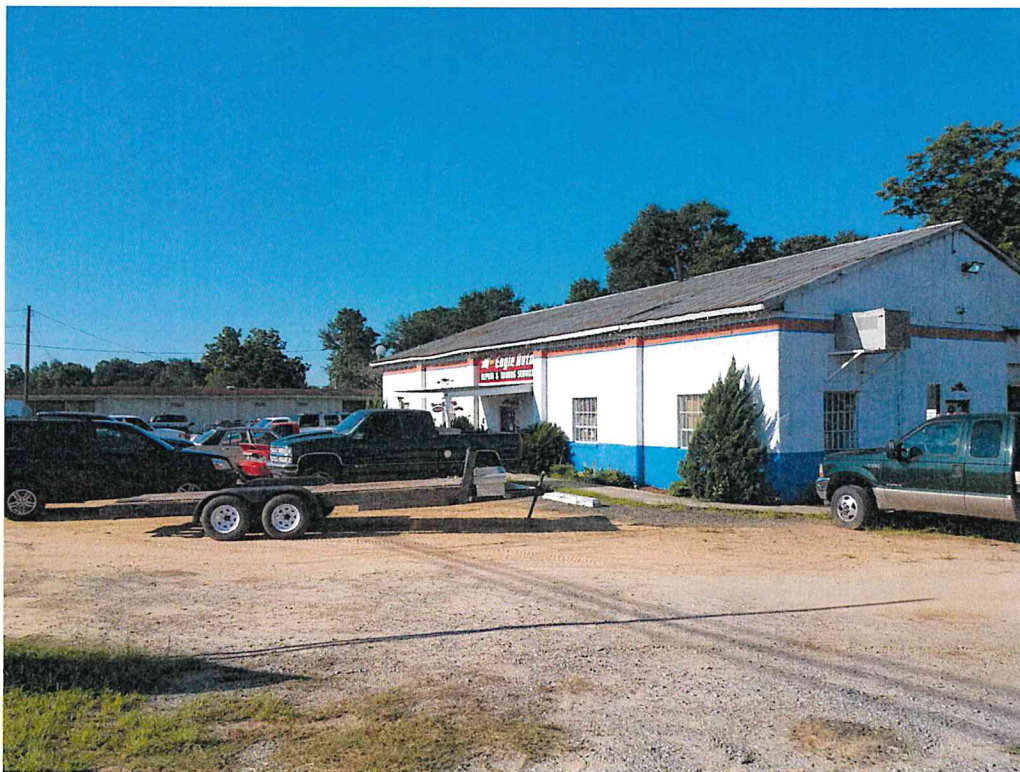
Picture 2 Subject Property Facing South
