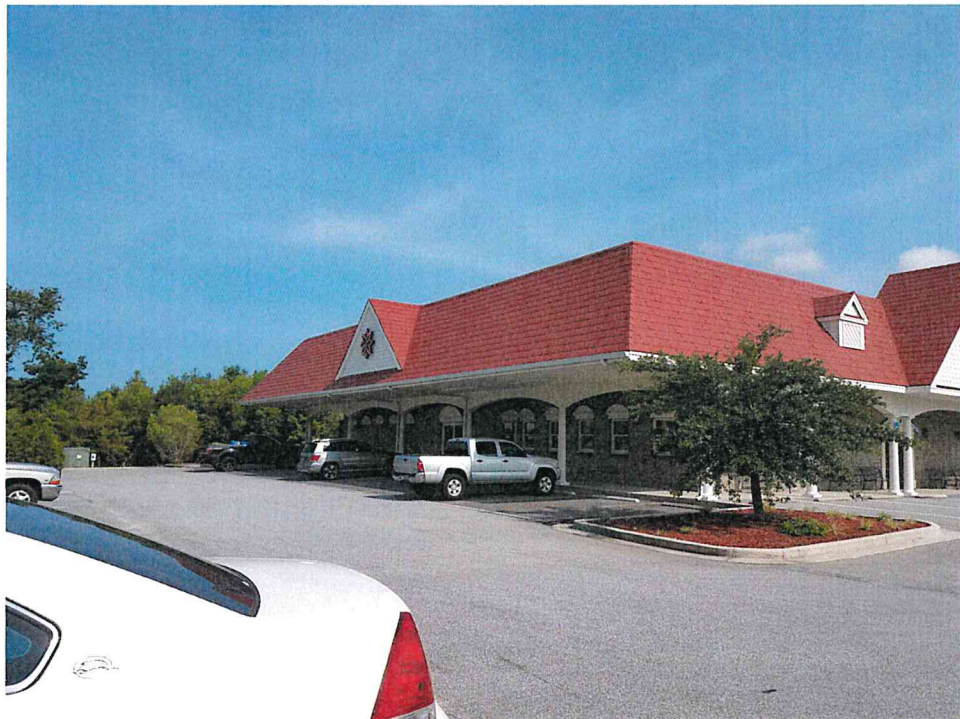
Picture 2: Southwest Facing Wall Depicting Installed Circular Logo Sign
