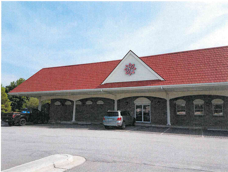
Picture 3: Southwest Facing Wall Depicting Installed Circular Logo Sign
