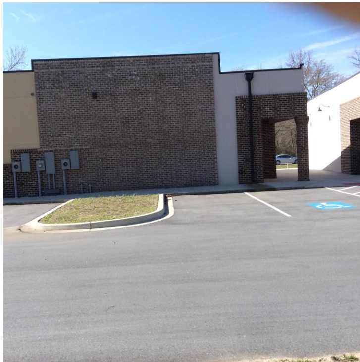
Picture 2: Back of Subject Site Facing South (one unit on the right side of the lot)
