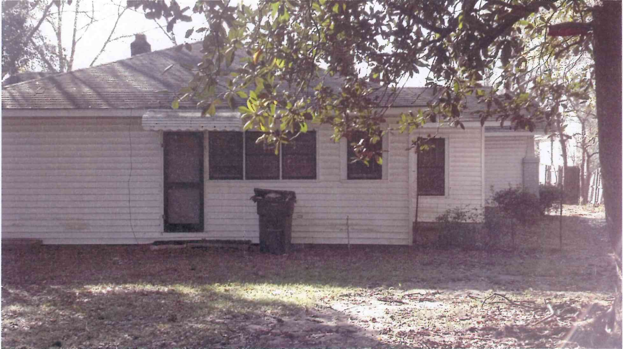
Figure 3: Rear of the building.
