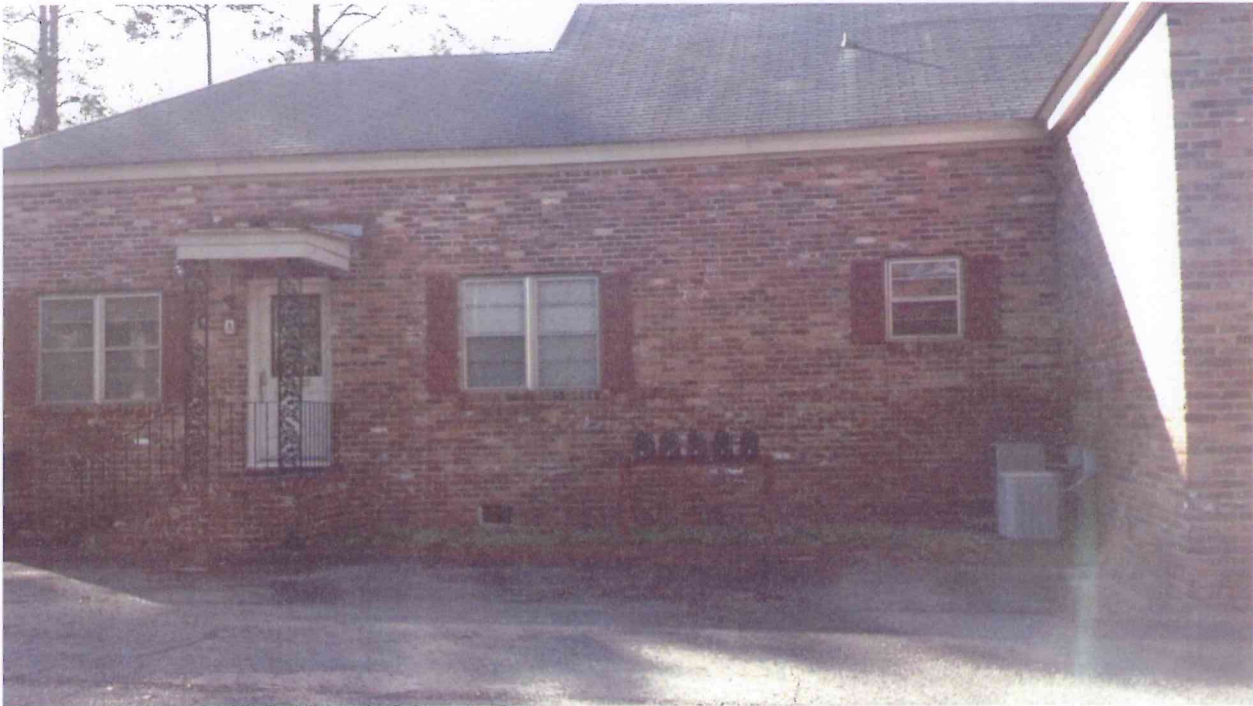
Figure 2: Side of the subject property.
