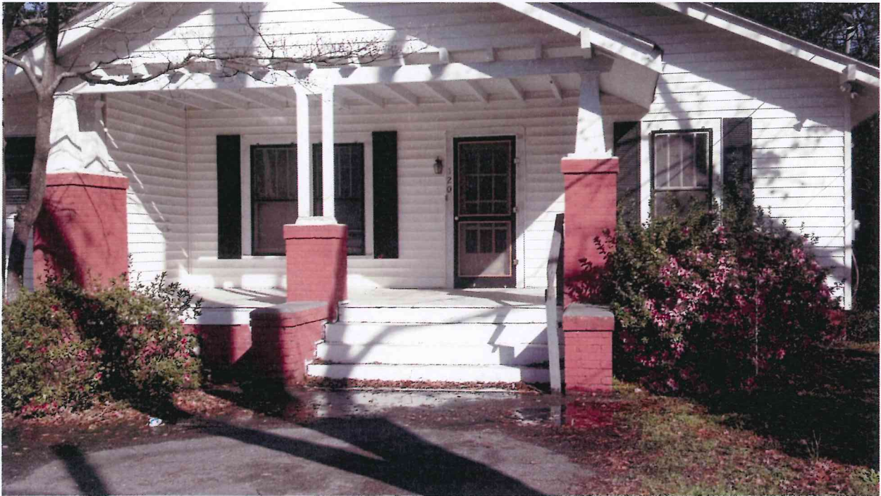
Figure 1: The Subject Property from North College Street.
