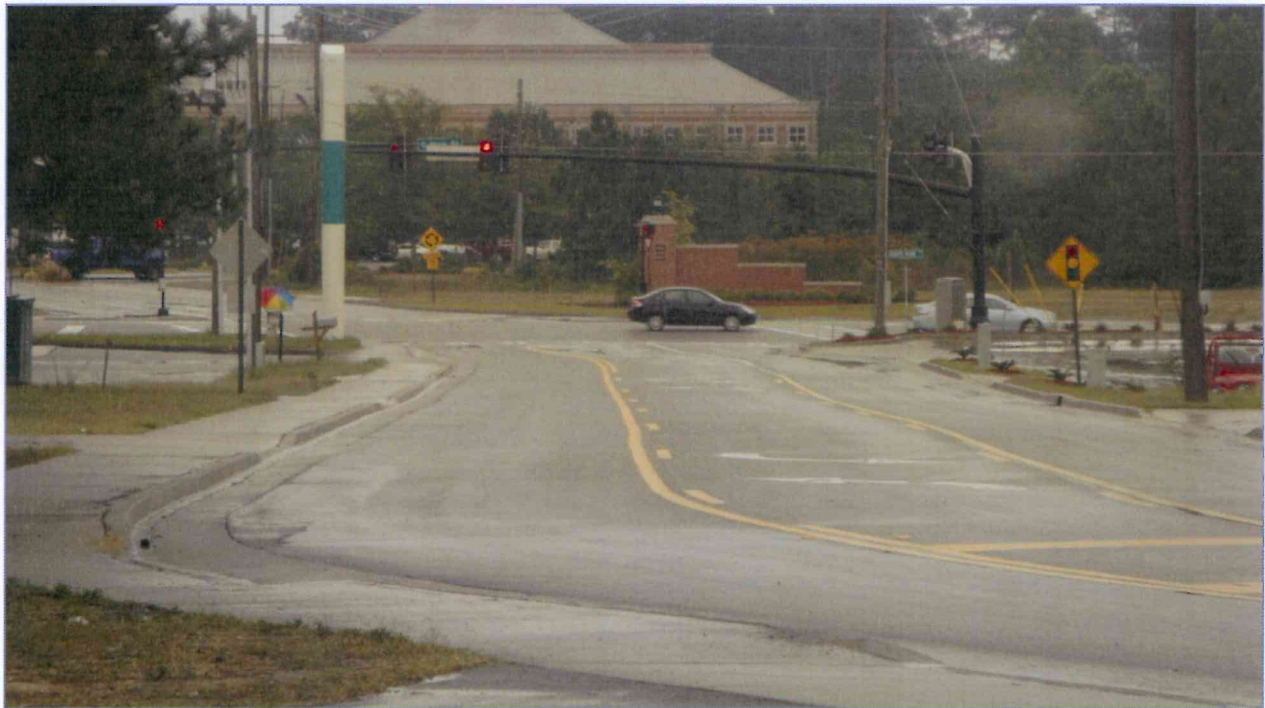
Figure 2: Intersection of Rucker Lane and Highway 301 South – viewed from Rucker Lane.
