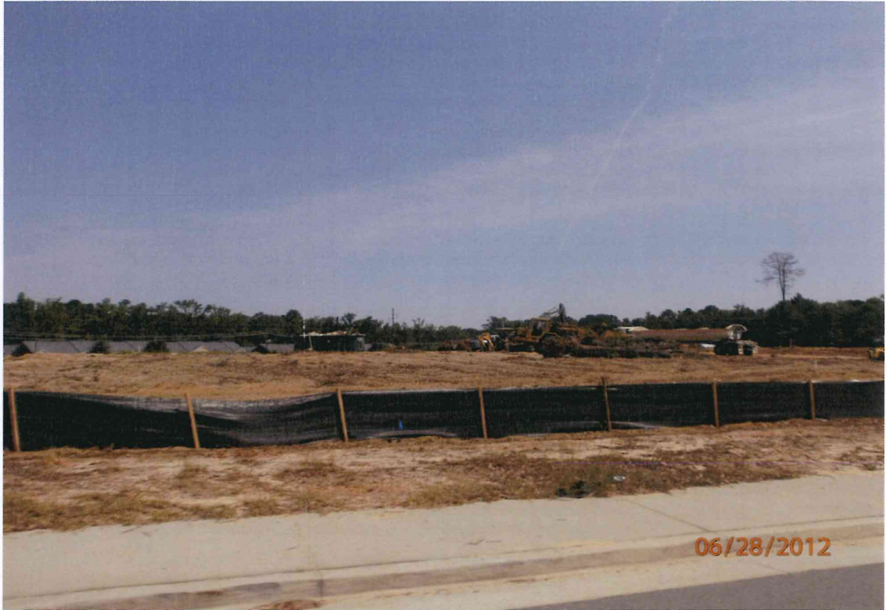
Figure 1: Subject Property – Under Construction.
