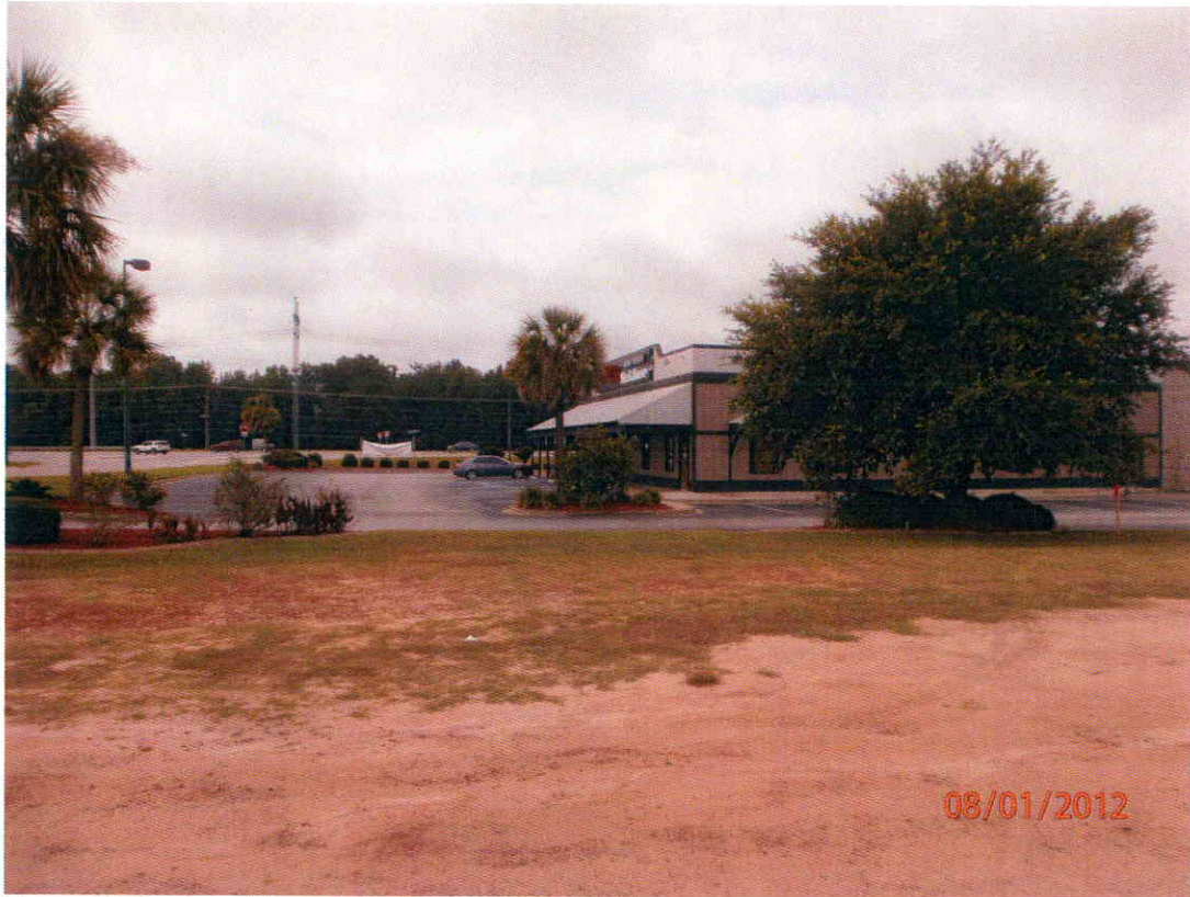
Figure 3: Southern Edge of the Subject Property facing Veterans Memorial Bypass.
