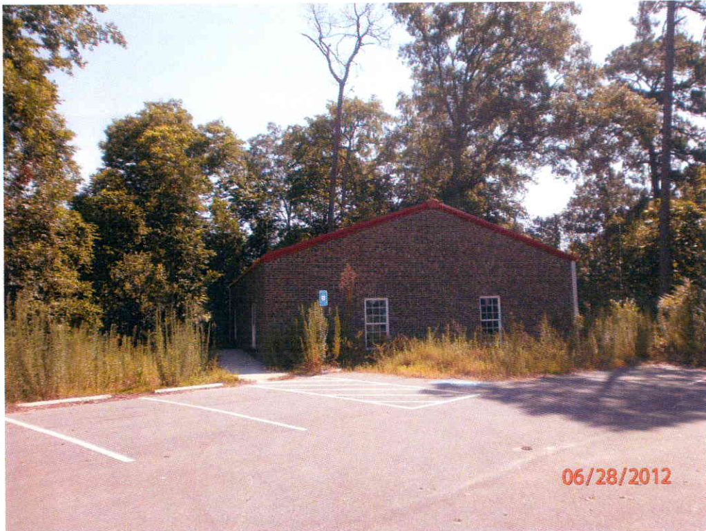
Figure 1: The Empty Incomplete Building Shell from North Zetterower Avenue.
