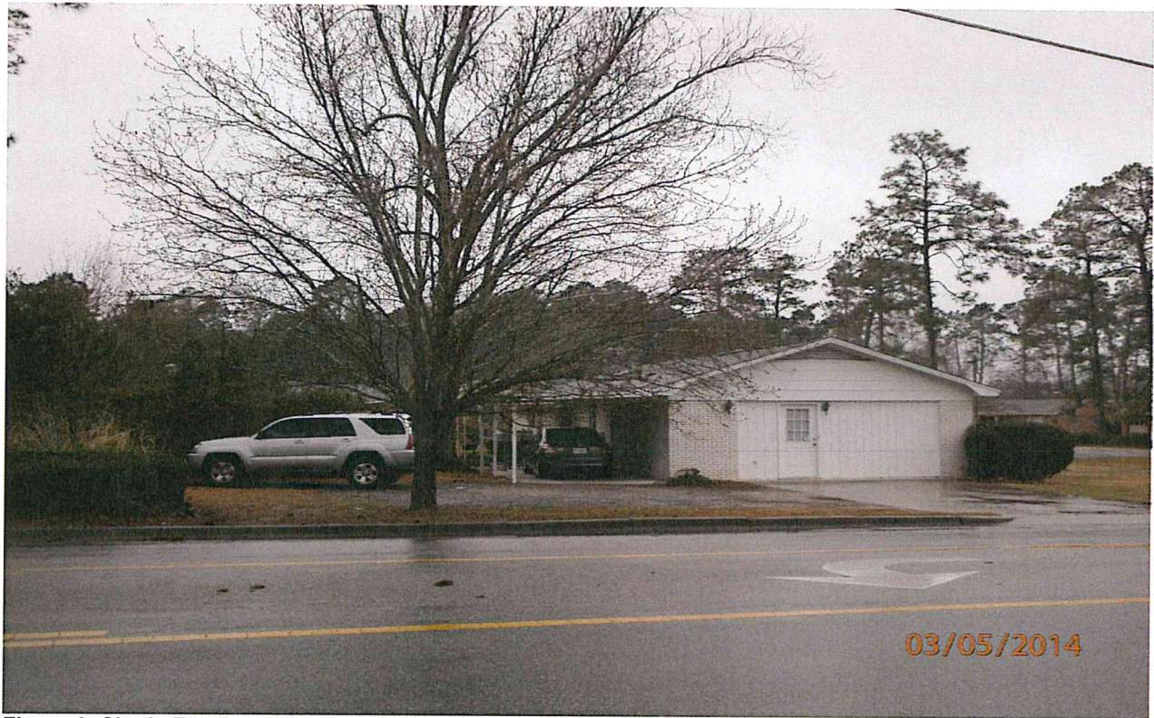
Figure 6: Single Family Homes across Gentilly Road from Subject Site.
