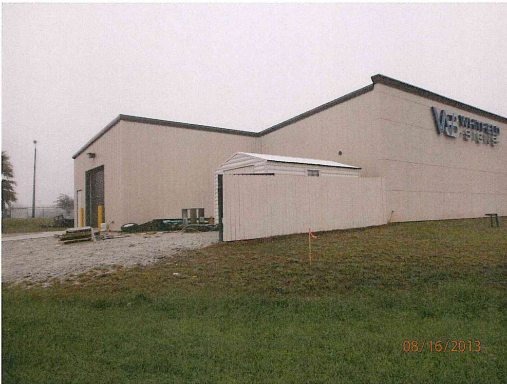
Figure 2: Subject Site rear northwestern view.
