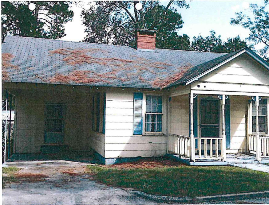
Picture 3 Rear of Subject Site
