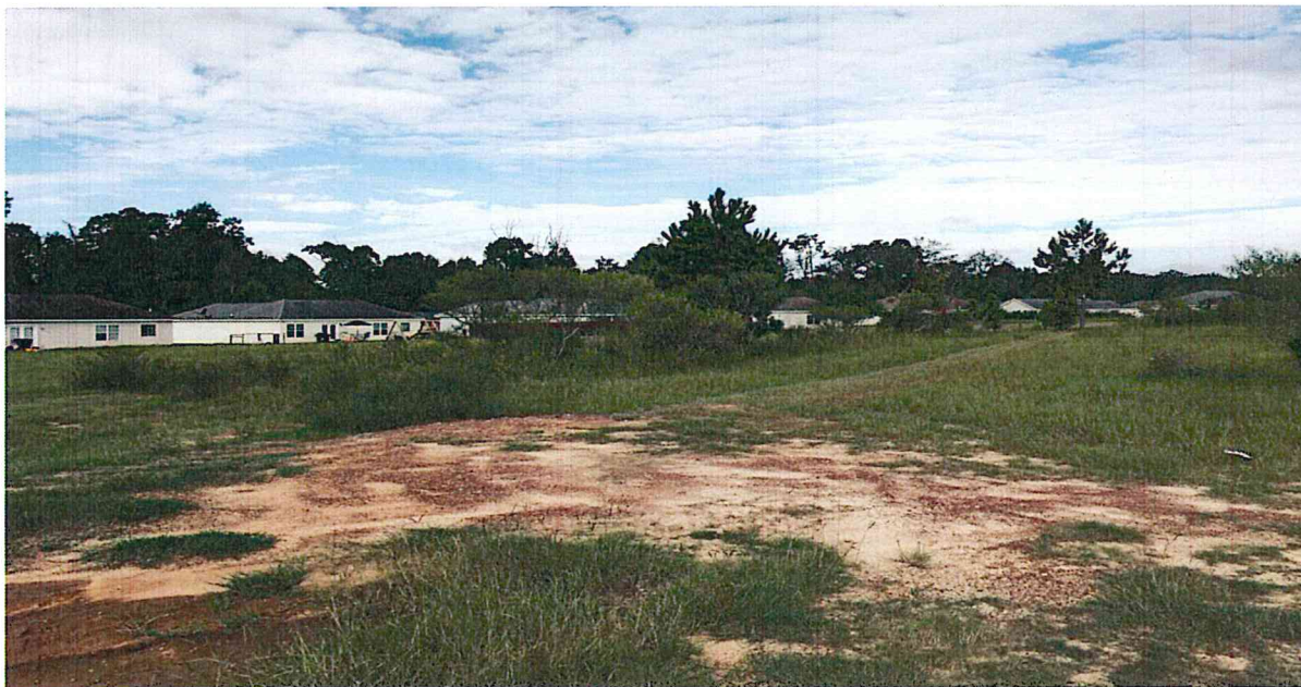
Drainage that runs along rear of Existing Lots 59- 47 & Proposed Lots 98 -110, Ph II
