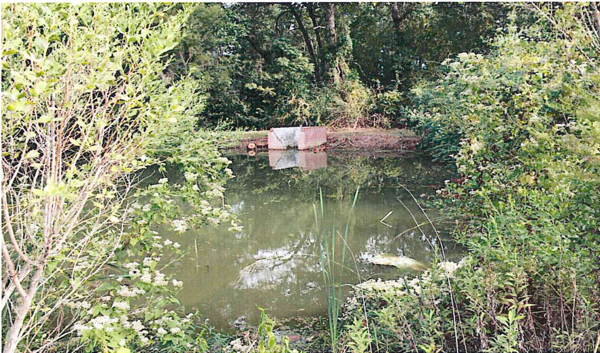
Detention Pond & Drainage/Whispering Pine Blvd between existing Lots 217 & 218
