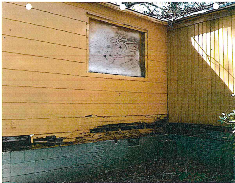
Picture 6 Rear of Subject Site
