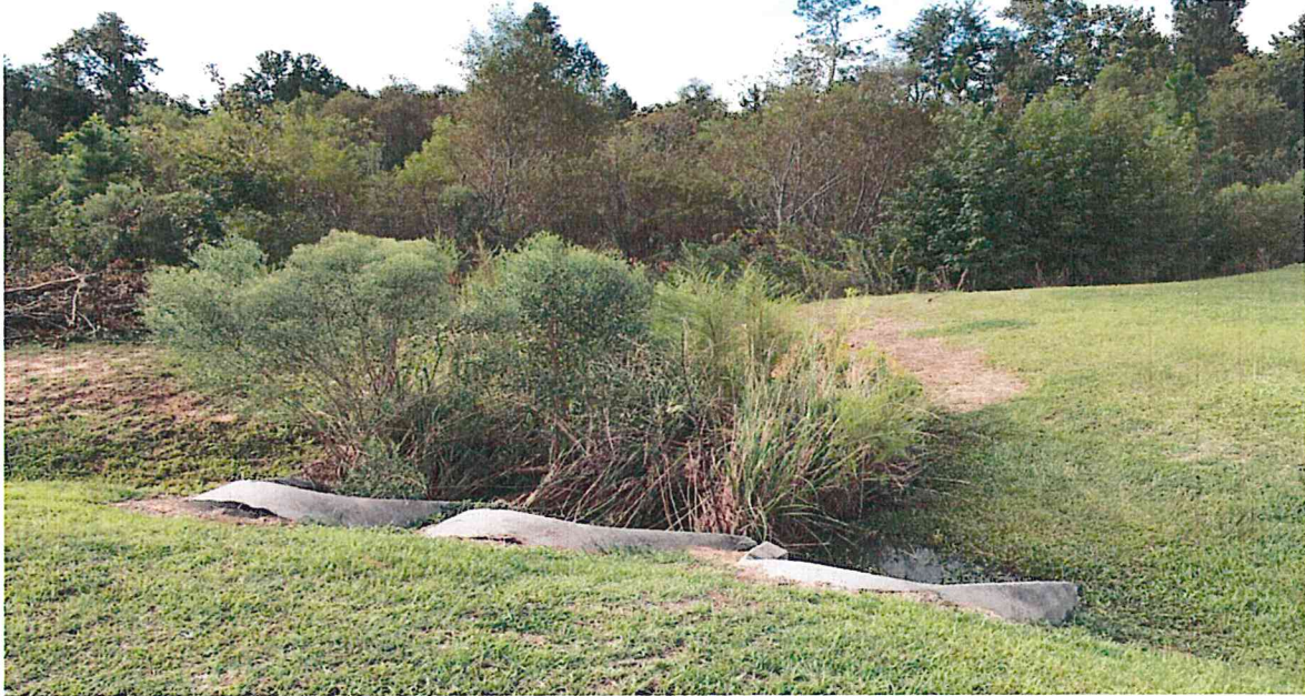
Detention Pond & Drainage located on Scotch Pine Ave between Lots 22 & 23
