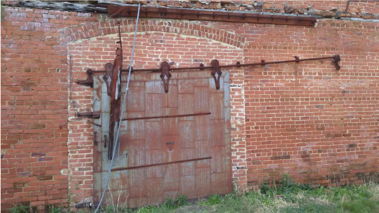
Picture 6 Exterior Entrance Depicting Masonry and Arched Doorway
