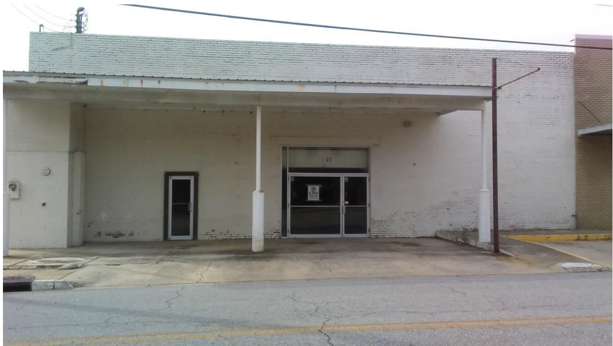
Picture 2 Exterior of 22 East Vine Street
