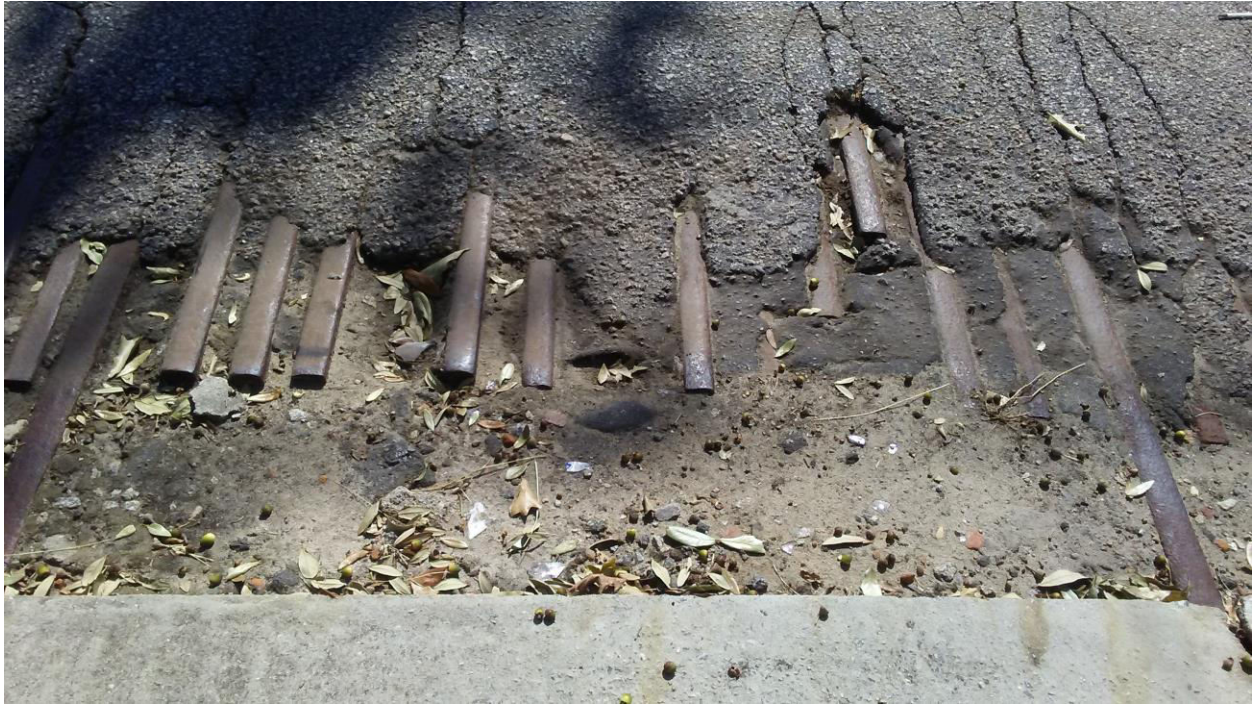
Picture 7 Railroad Ties Located across East Vine Street belonging to Central of Georgia Railway
