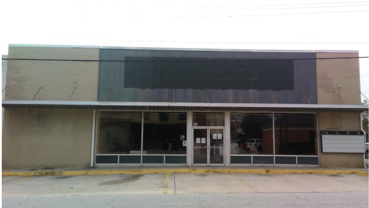
Picture 1 Exterior of 20 East Vine Street, the Former Smith Supply Co.
