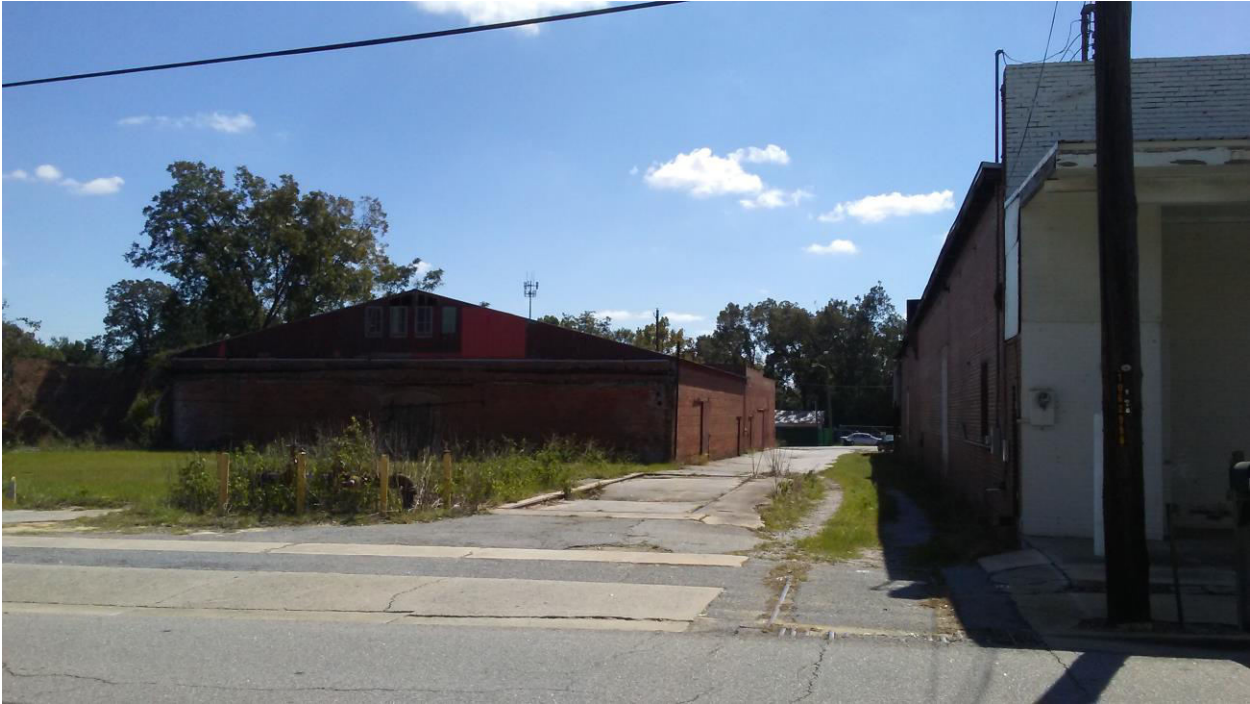
Picture 3 Exterior Depicting Central of Georgia Railway Easement
