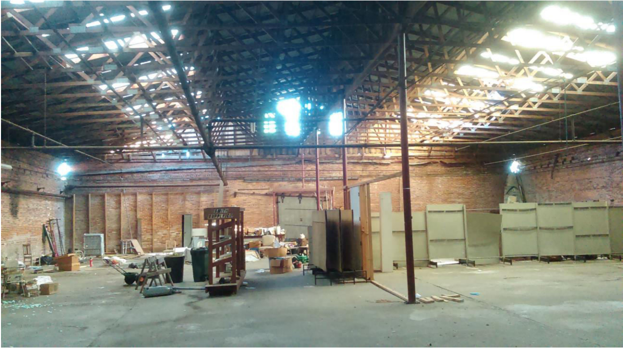
Picture 11 Interior Depicting Exposed Brick and Succession of Skylights
