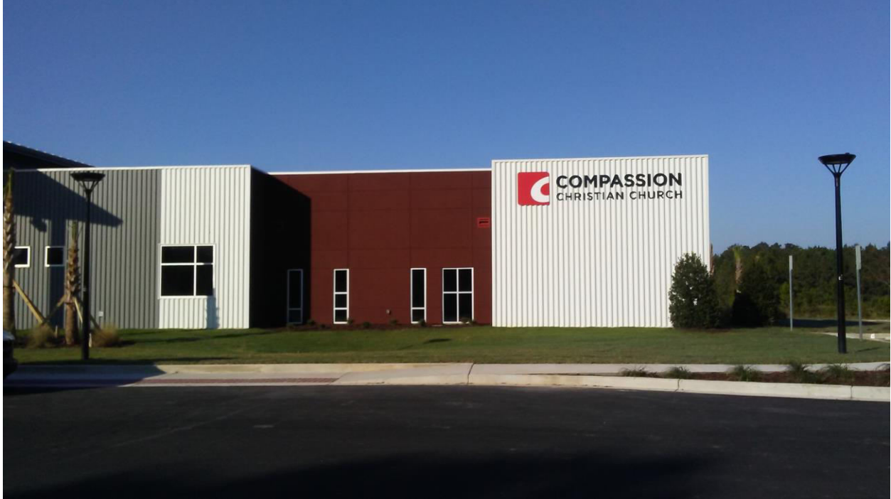
Picture 1 Installed Building Sign at 73.35 Square Feet
