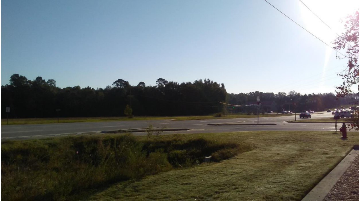
Picture 9 Subject Site from Parking Lot of Family Dollar across Veterans Memorial Parkway
