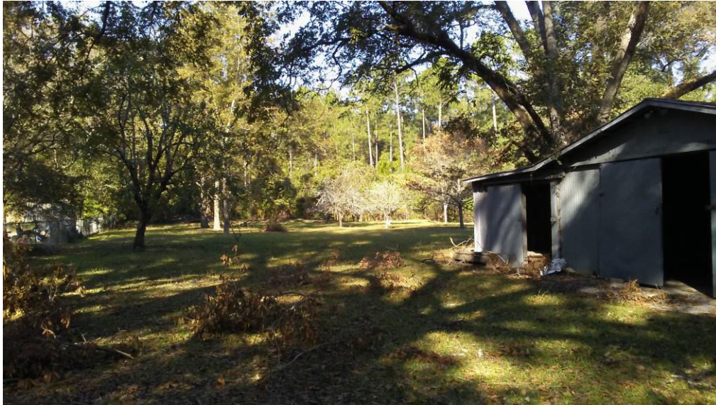
Picture 7 Existing Structure at Rear of Property
