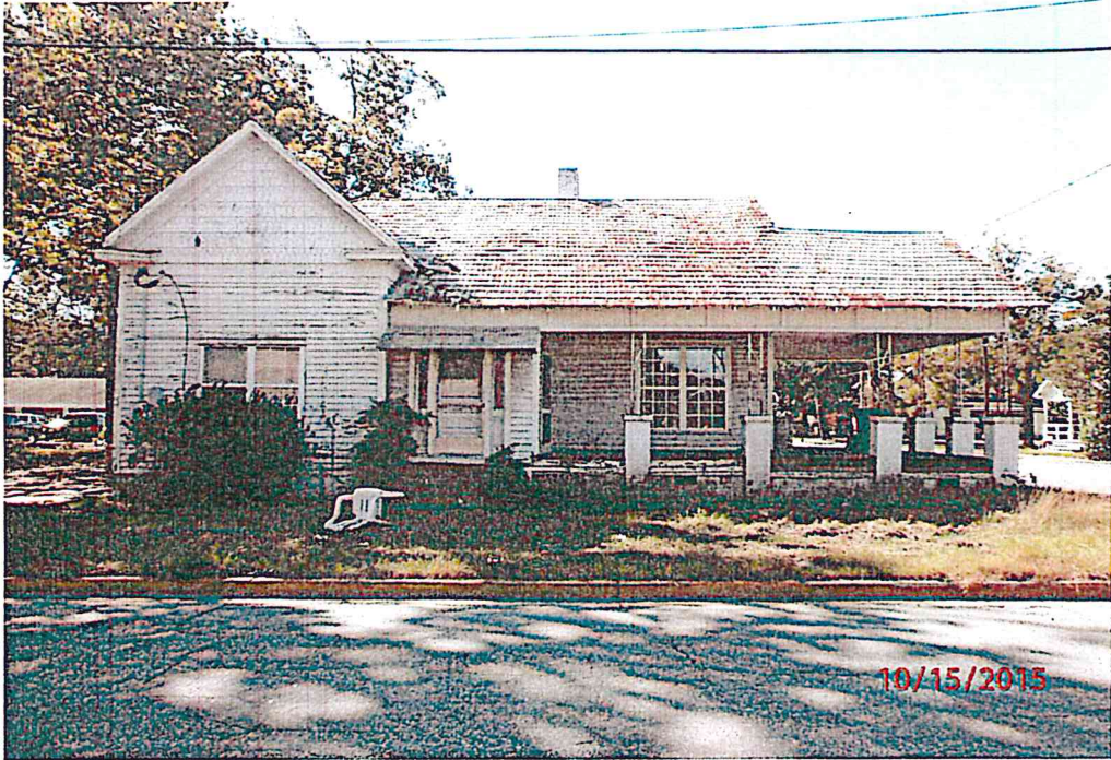
Picture 3 Side of Tax Parcel S19 000050 000 Facing West (Demolition Request)
