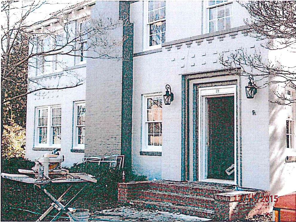
Picture 1 Tax Parcel S19 000032 000 (12 Bulloch Street) Facing Southeast (5 bedrooms)
