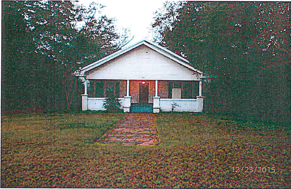
Figure 1: The Subject Property from Broad Street
