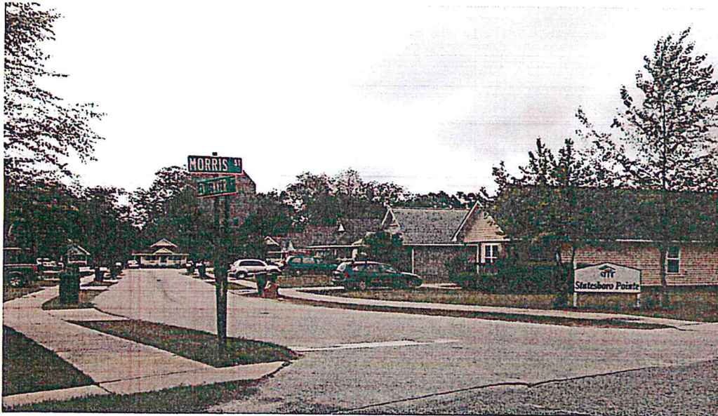
Photo 4: Planned Unit Development that is directly Adjacent to the above Photo.
