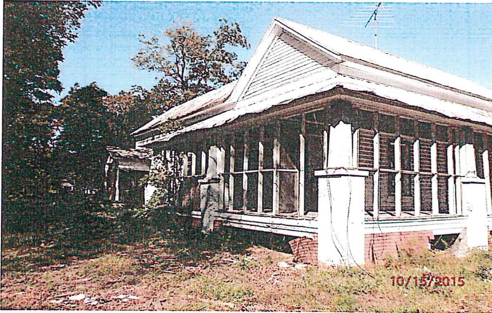
Picture 3 Subject site facing northwest (left side of structure)
