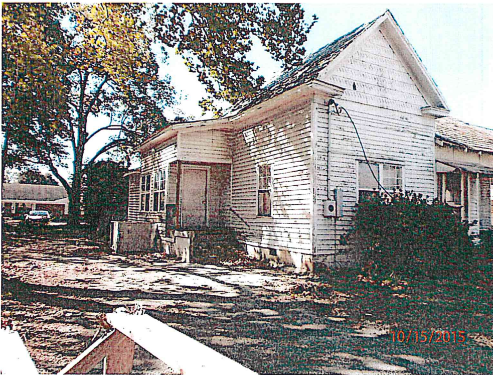
Picture 2 Back of Tax Parcel S19 000050 000 Facing West (Demolition Request)
