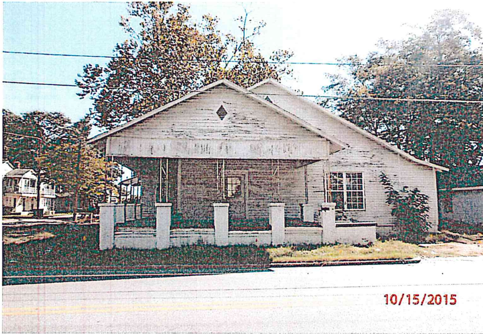
Picture 1 Tax Parcel S19 000050 000 Facing East (Demolition Request)
