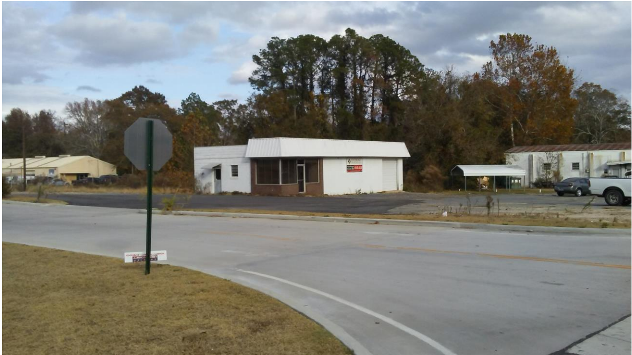
Picture 2 Subject Site Facing East Depicting the Vacant Structure on the Lot
