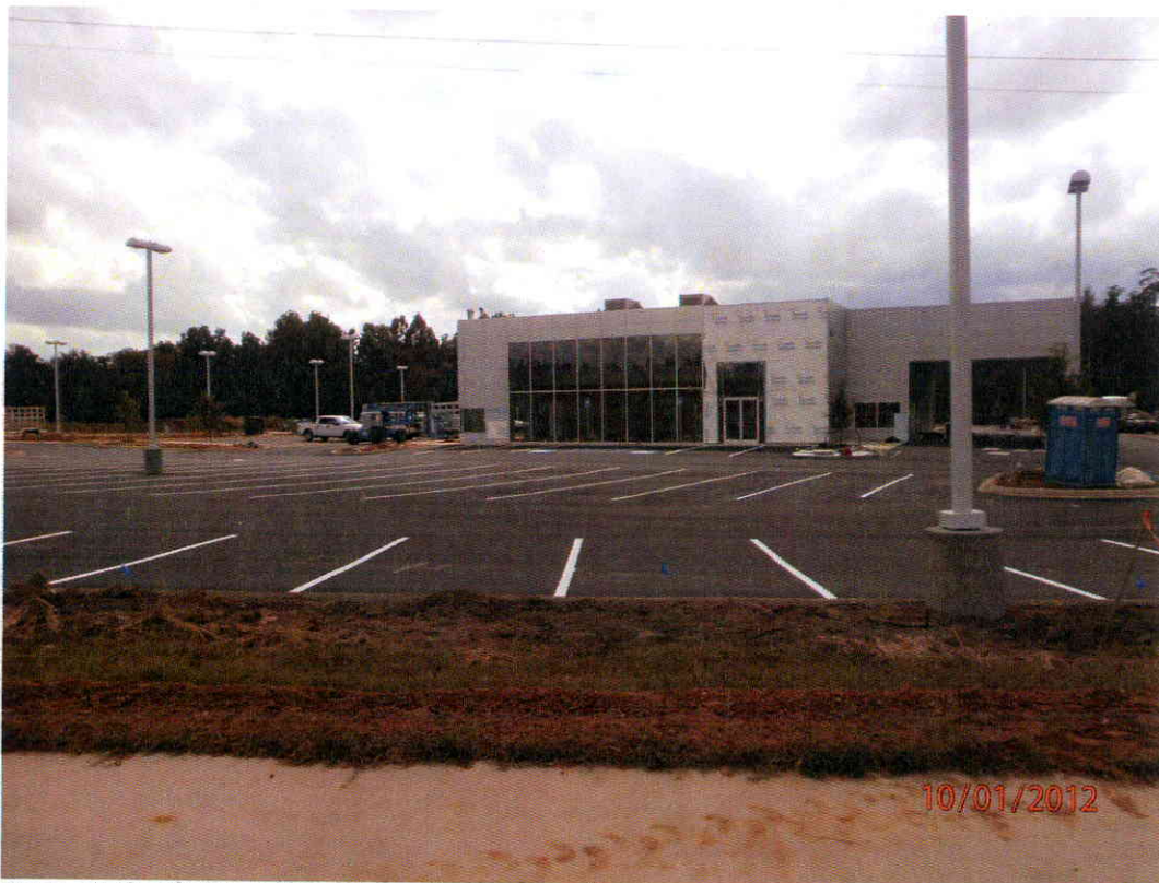
Figure 2: The Subject Property under Construction from Brannen Street.
