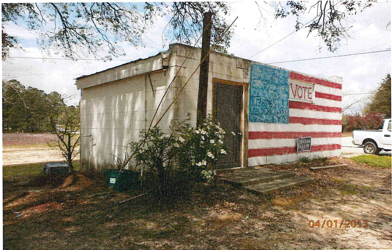
Figure 3: Rear of the subject site.
