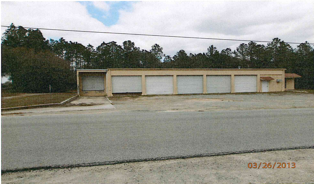
Figure 5: Storage facility across Fletcher Drive from Subject Site.
