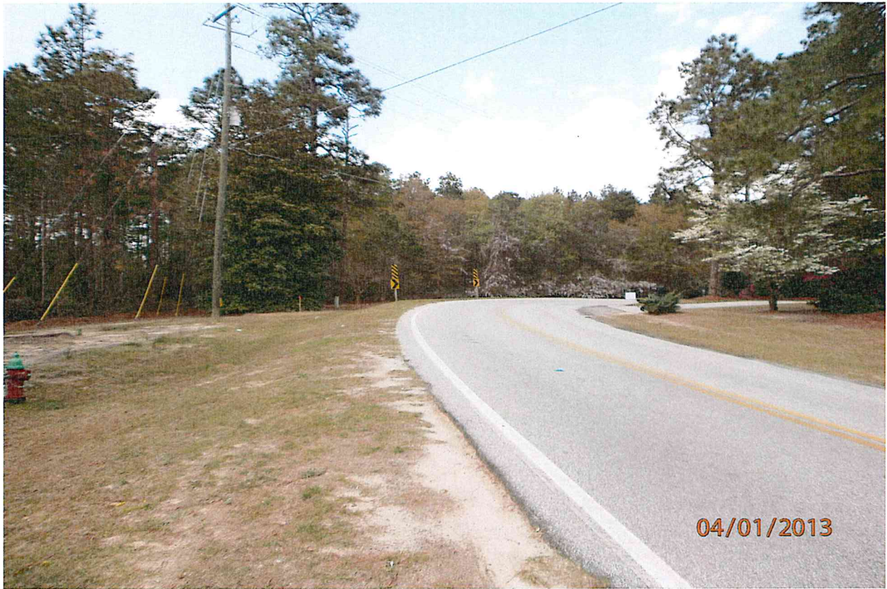
Figure 5: Cawana Road to the North of the Subject Property.
