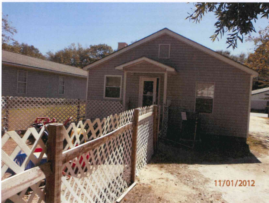
Figure 4: View of the back of the building.
