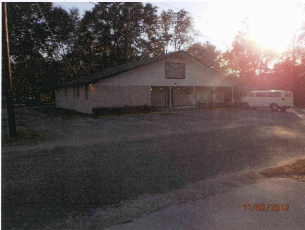
Figure 6: Mortuary to the southwest of the Subject Site across James Street.
