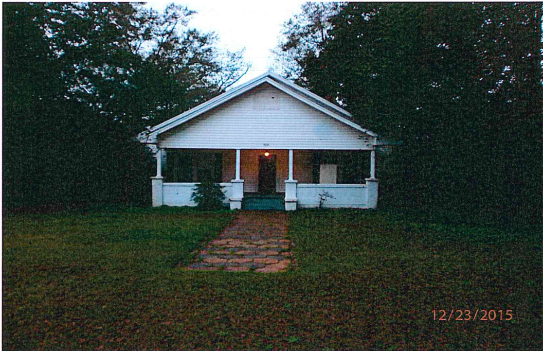
Figure 1: The Subject Property from Broad Street
