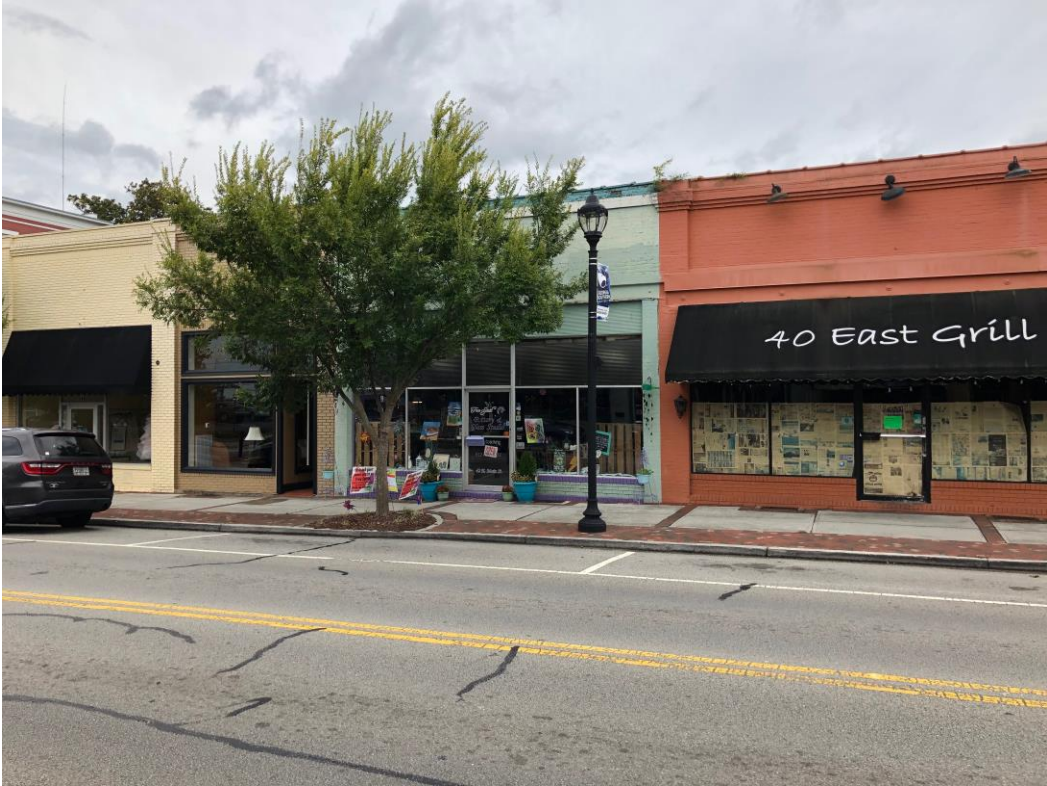
Picture 3: View of the abutting properties to the east on East Main Street, specifically Free Spirit Pottery & Glass Studio.
