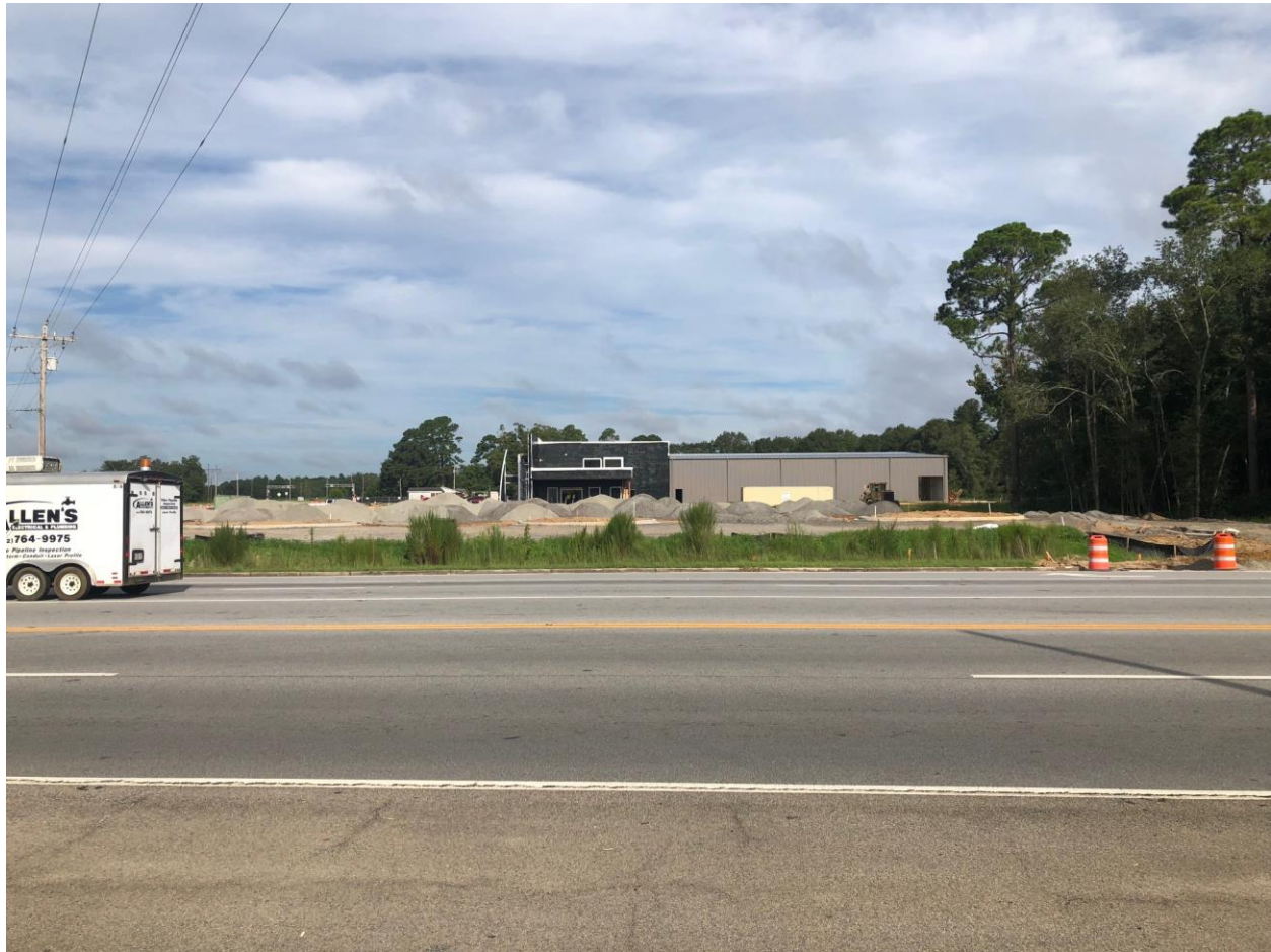
Picture 7: View of the surrounding property to the west of the subject site, currently new construction site for JC Lewis Ford Car Dealership.
