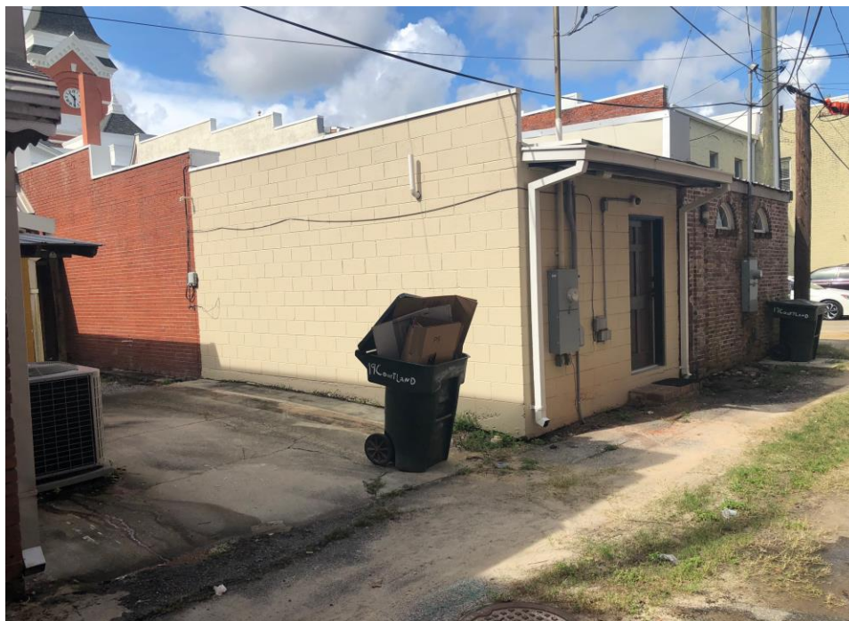
Picture 4: Looking southwest from the alley located to the rear of the subject site, the proposed expansion area for Divvy Desk
