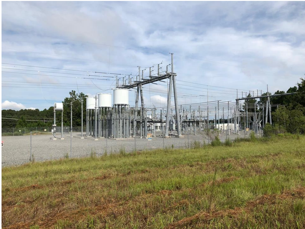
Picture 5: Looking north from the subject site, currently a Georgia Power utility substation located along the subject site's northern boundary
