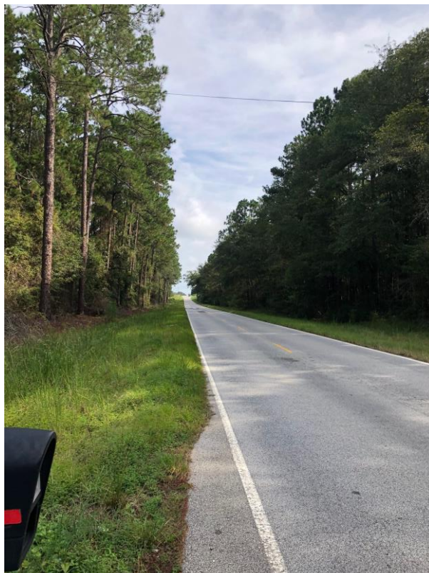
Picture 8: Looking north along Old Register Road, an additional view of the eastern boundary of the subject site.
