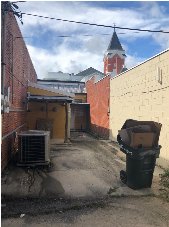
Picture 3: Looking south from the alley located to the rear of the subject, the proposed expansion area for Divvy Desk.
