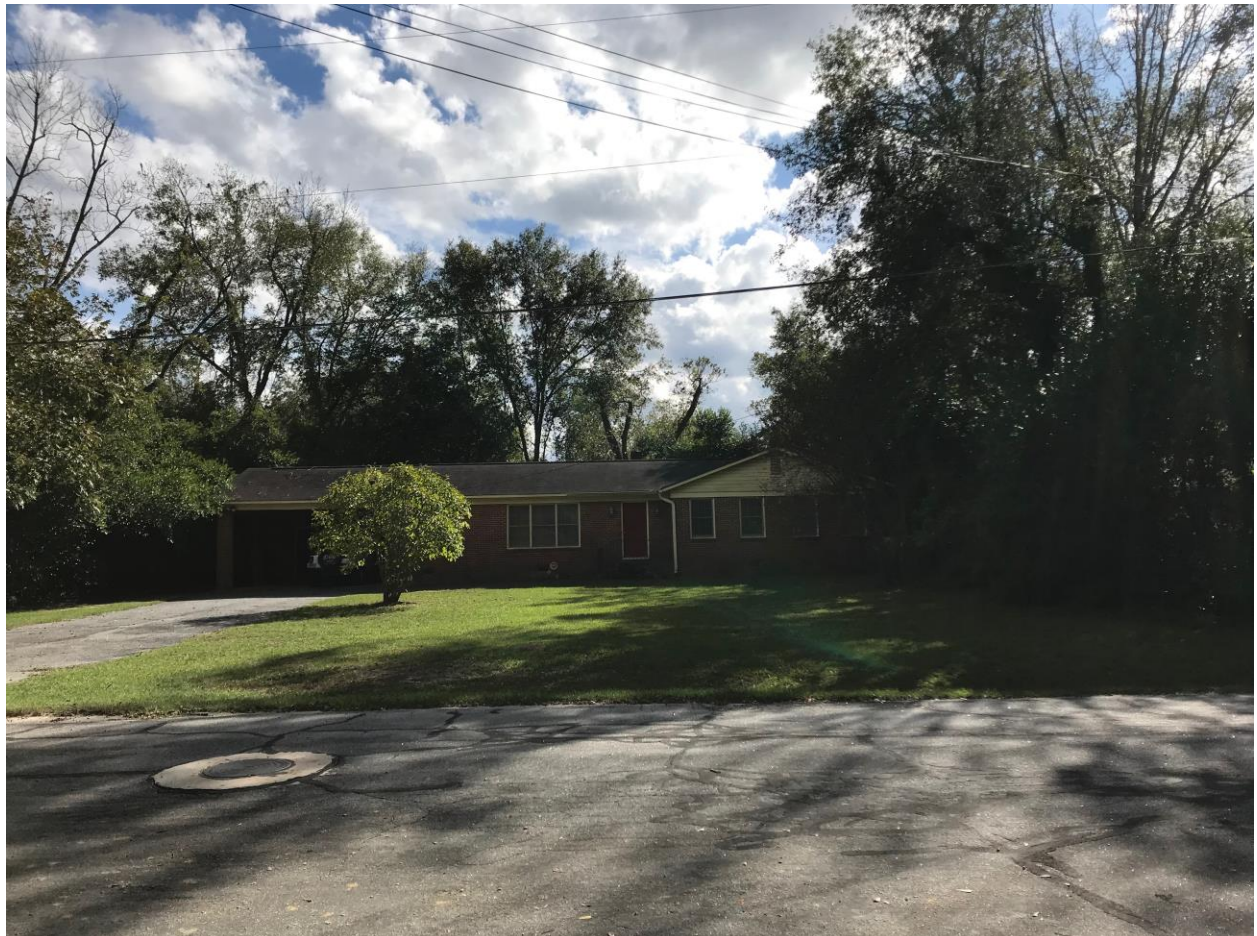
Picture 2: View of the subject property, looking north from Niver Road.
