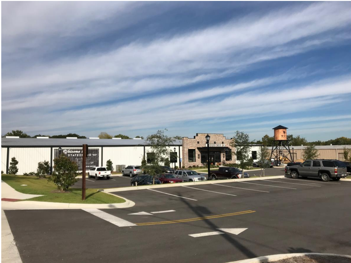
Picture 5: Looking west from the subject site, the Whitfield Signs Office/Warehouse Building.
