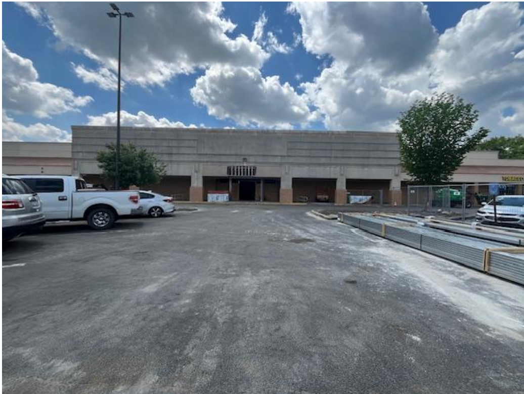
Subject property: view of the building and take note of significant size of the building.
