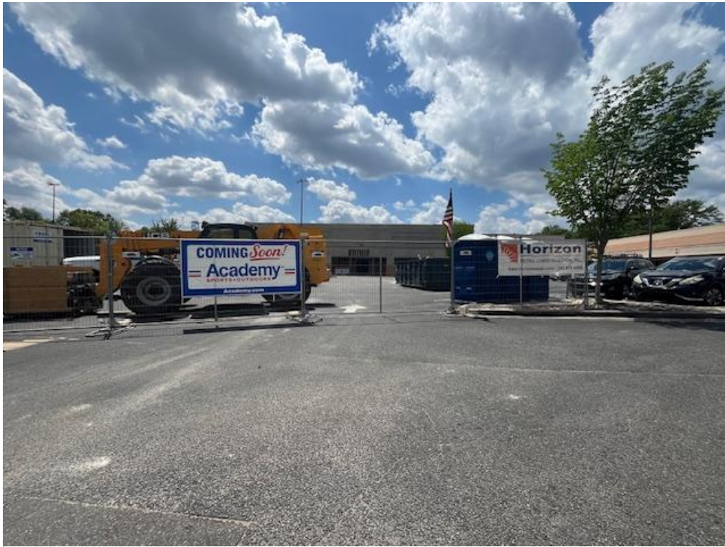
Subject Property: view of the property from the parking lot along the ROW on East Northside Drive, facing west.
