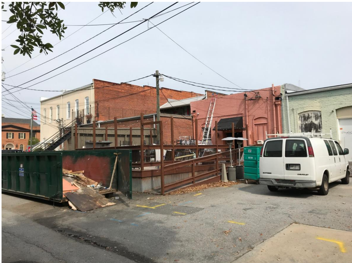
Picture 2: Rear view of subject site, looking north from Anderson Alley. Also, a view of the existing deck prior to the renovations being requested under CBD 19-04-01 .
