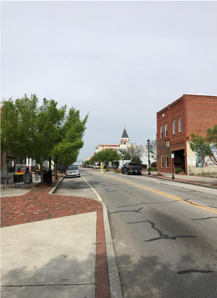
Picture 3: Looking west down East Main Street, a view of the adjacent properties and downtown area near the subject properties.
