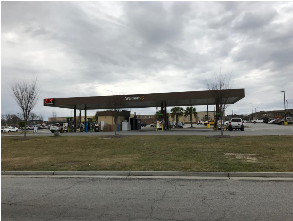
Picture 3: View of the adjacent property to the east of the subject property, currently Walmart Gas Station.
