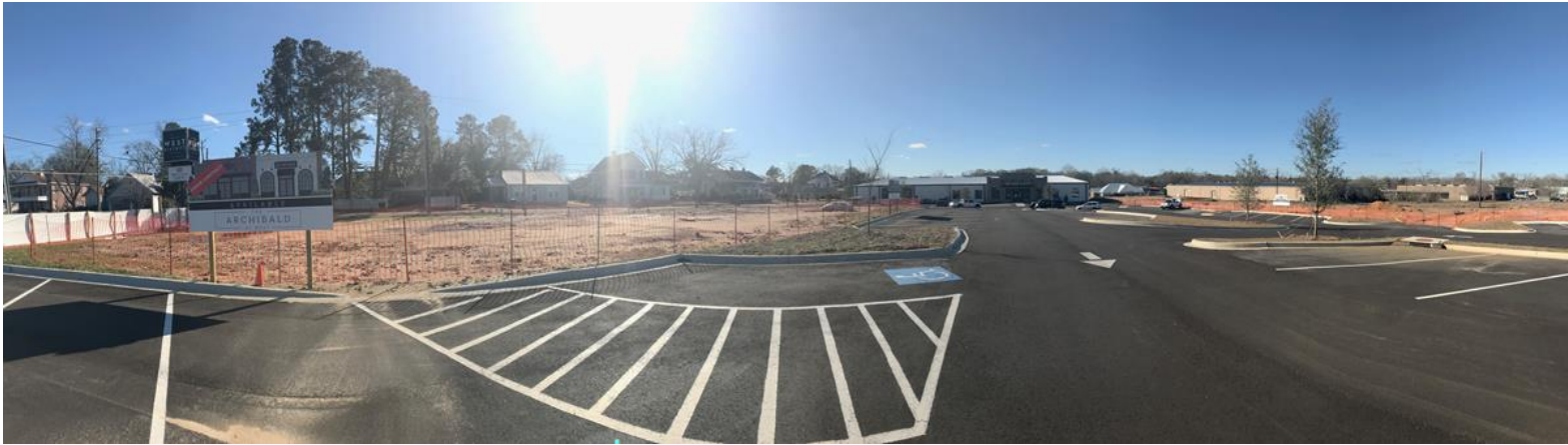
Picture 3: View of the adjacent properties to the south of the subject site, currently the West District Development Phase I vacant parcels and the Whitfield Signs Building.
