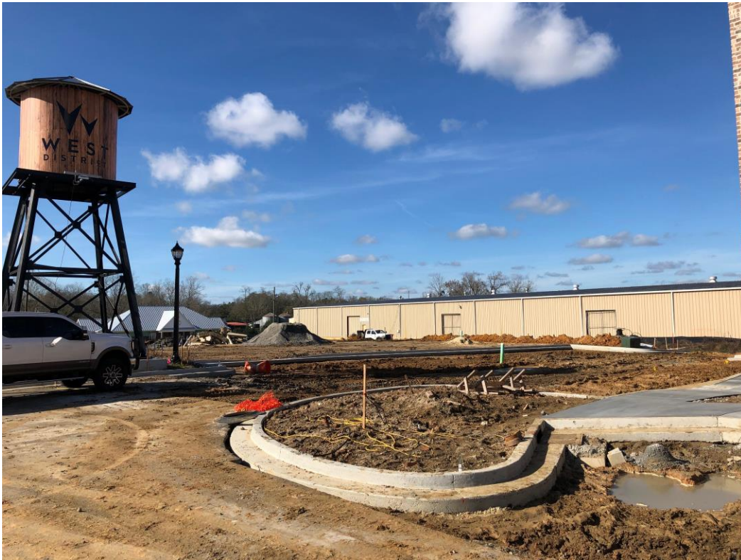
Picture 3: View of the adjacent properties to the east of the subject site, currently under construction.
