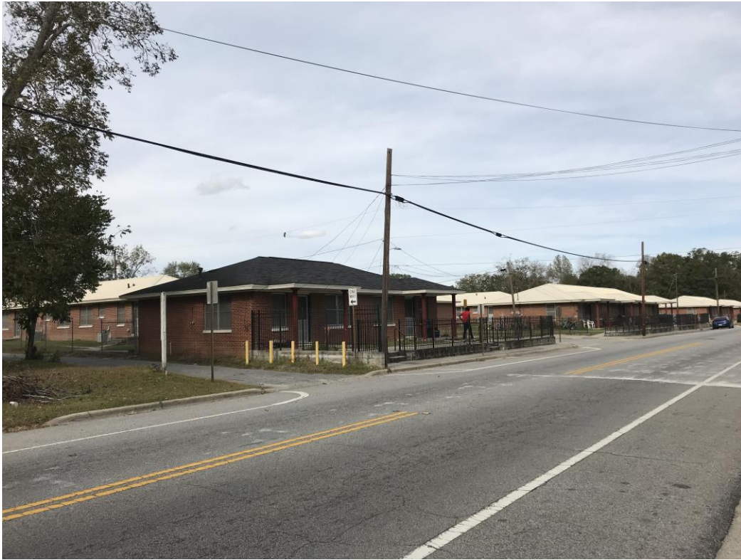
Picture 7: View of surrounding properties to the northeast of the subject site, currently Butler Homes Apartment Community.
