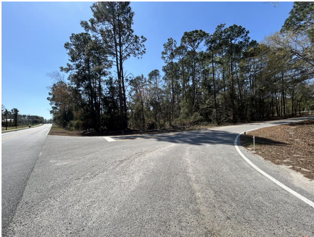
Subject property: Tract 2 from the ROW on Packinghouse Road, facing south.
