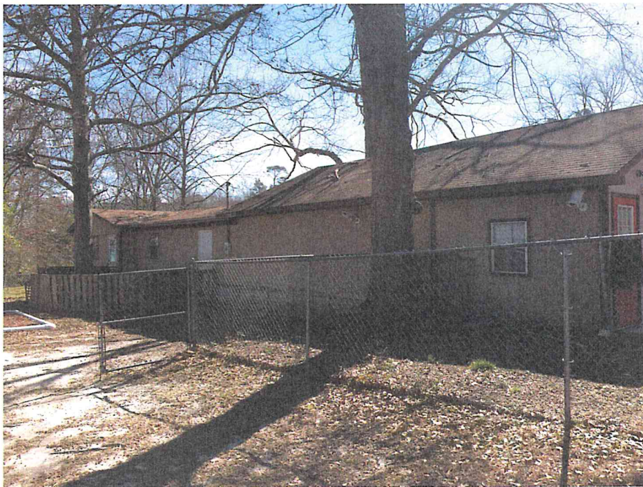
Picture 8 Subject Site Facing East Depicting Rear Elevation
