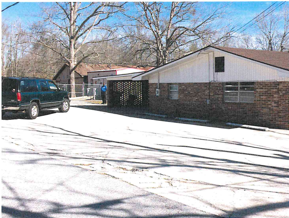
Picture 4 707 West Jones Avenue facing North East Depicting Portion of the Parking Lot
