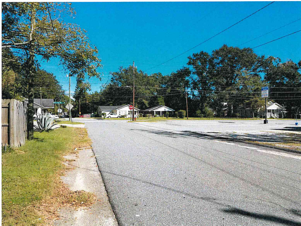
Picture 3 Roundtree Street Facing Martin Luther King, Jr. Drive
