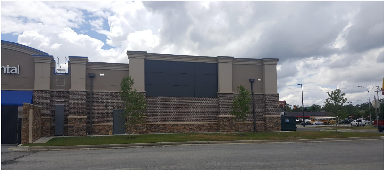
Picture 4: Installed signed for businesses in close proximity to the applicant, looking north from the rear elevation.
