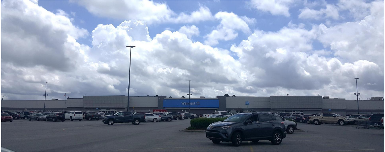
Picture2: Subject Site depicting proposed location for additional signage (orange section), right side of front elevation.
