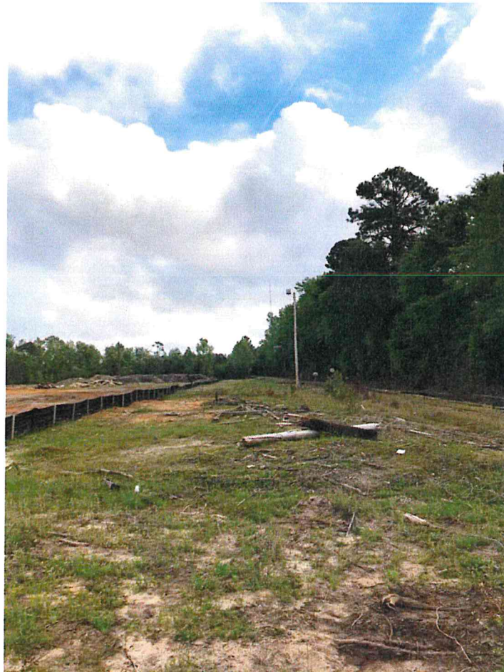
Picture 3: View of the subject property, looking west along the subject site's rear property line boundary.
