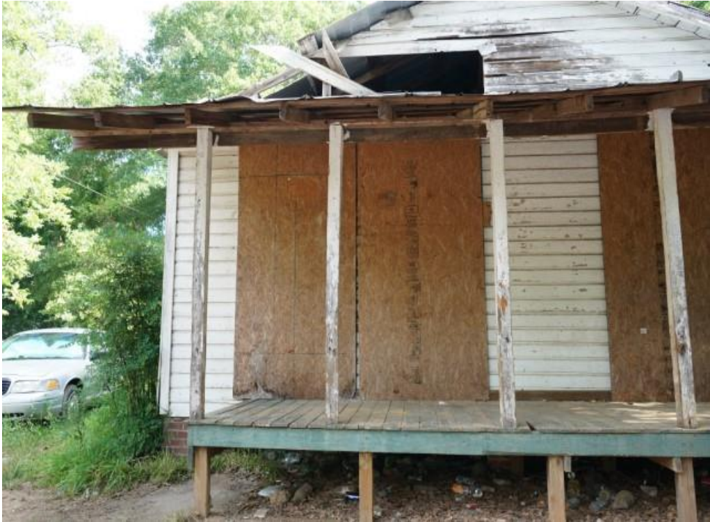
Vacant and Dilapidated Home on Inman Street - Johnson Street Neighborhood
