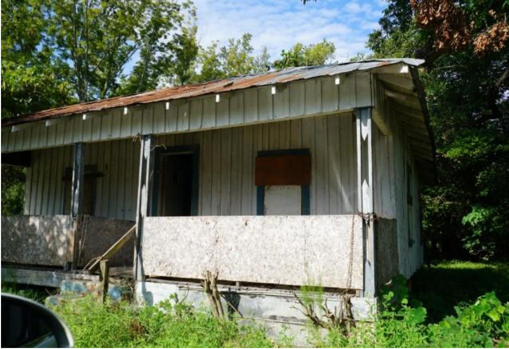
Vacant and Dilapidated Home on Rackley Street – Johnson Street Neighborhood
