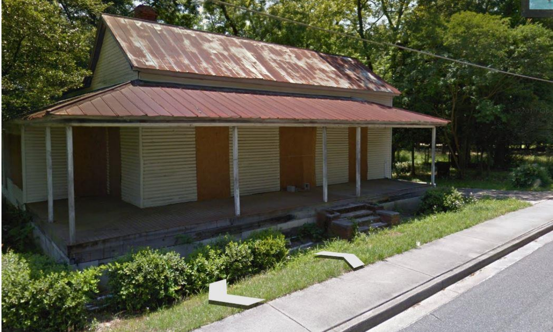
125 Morris Street – Rehab House
