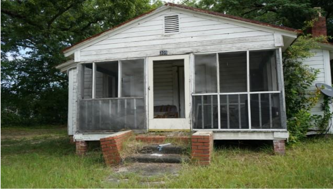
Vacant Dilapidated Home in MLK Neighborhood
