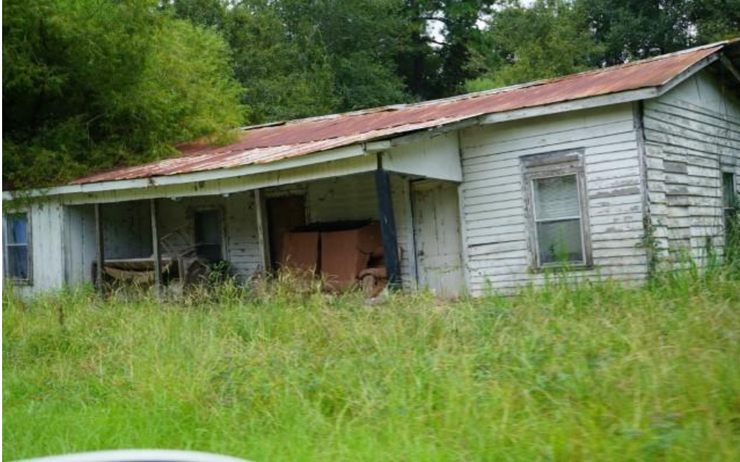
Vacant Dilapidated Home in Whiteville Neighborhood
