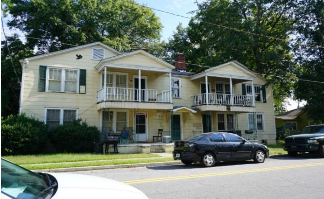
Substandard Apartment Structure Adjacent to The Blue Mile Corridor Johnson Street Neighborhood
