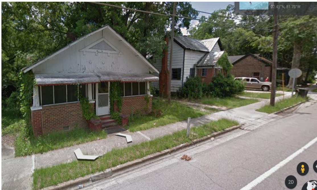
215 Johnson Street – Rehab House
