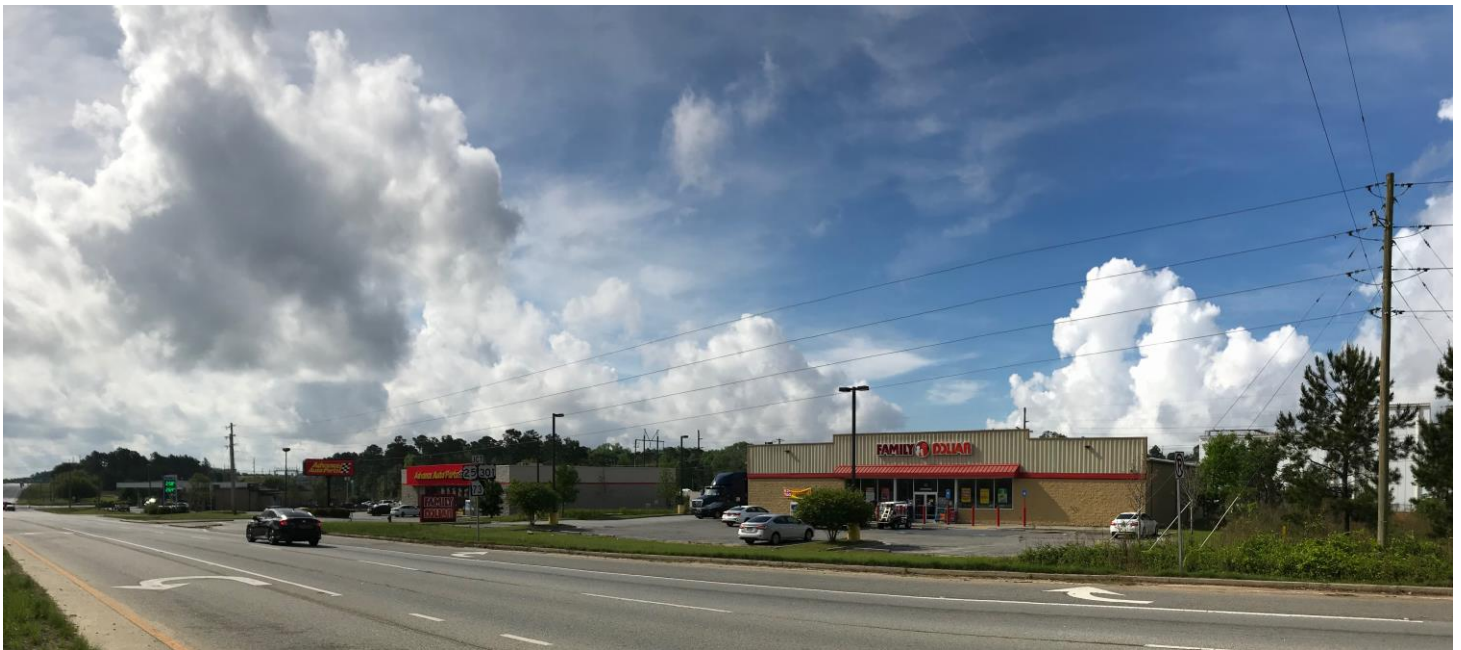
Picture 6: Looking southwest from the subject site, currently commercial retail – Family Dollar Store, Advanced Autoparts, and other commercial retail uses.
