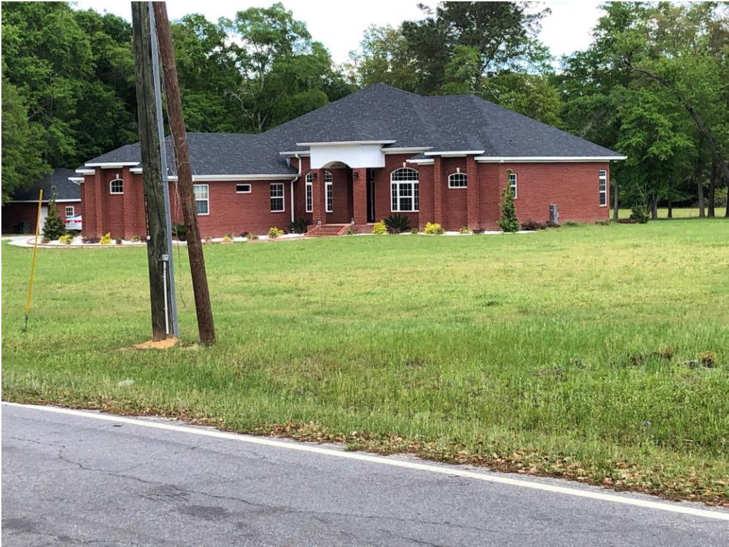
Picture 4: View of the adjacent property to the northeast from the corner of Christie Lane and Francis Scott Drive.
