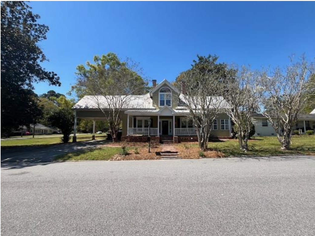
Subject Property: view of the property from the ROW on Park Ave, facing west.
