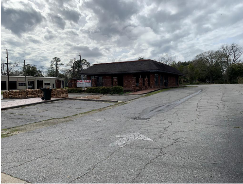
Picture 1: Looking west from South Main Street, a view of the subject site, currently a vacant restaurant building.
