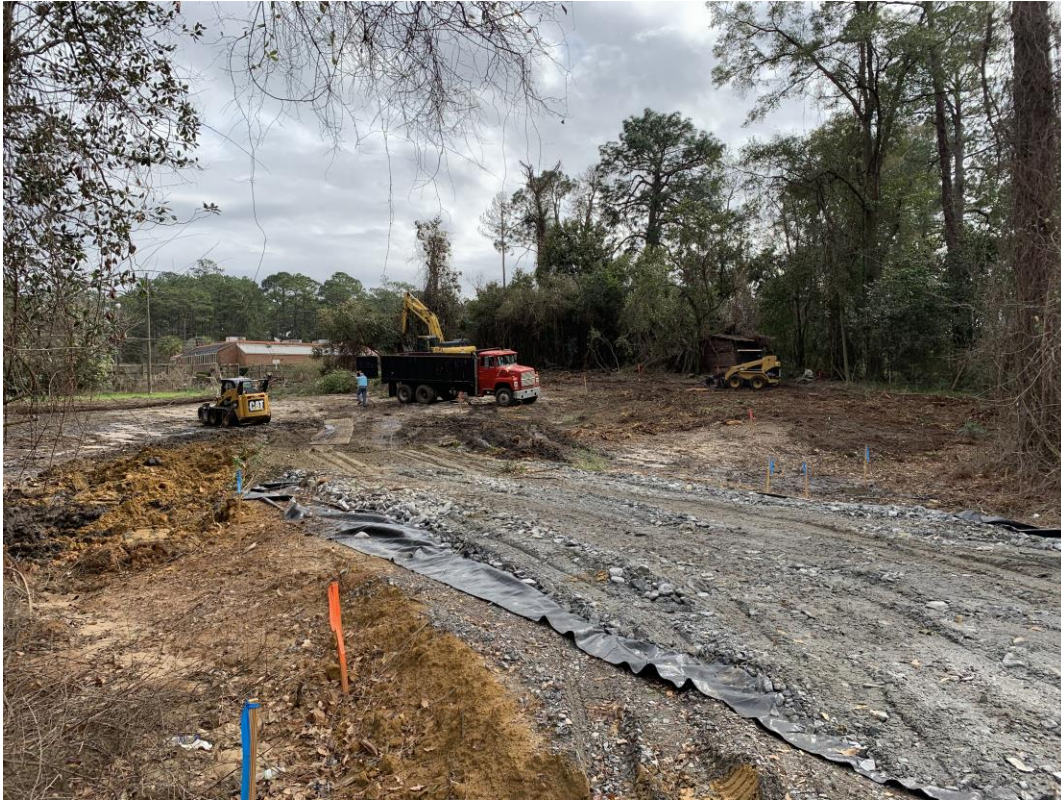
Picture 1: Looking east from South College Street, a view of the subject site, currently an active construction site for the new Hidden Hollow apartment community.
