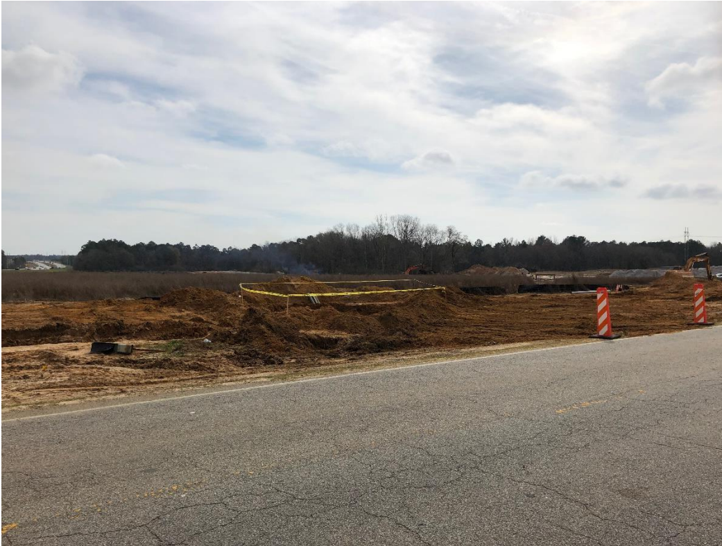
Picture 3: General view of the site, currently under construction, from Old Register Road
