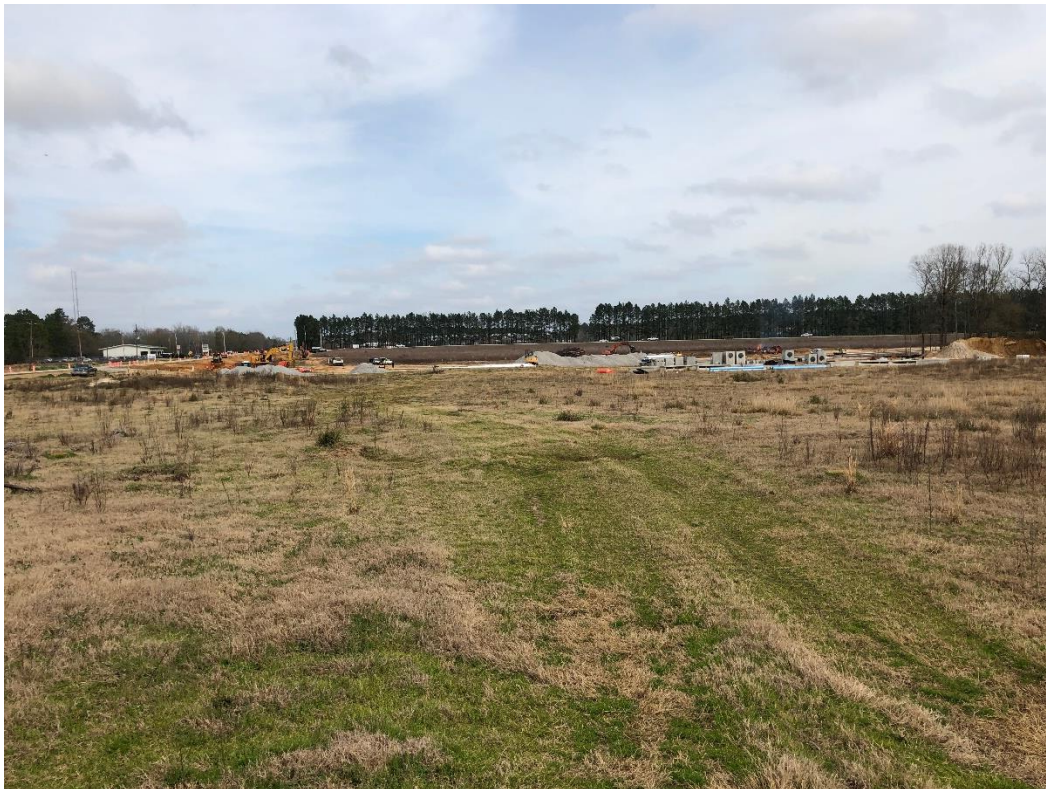
Picture 4: General view of the site, currently under construction. .
