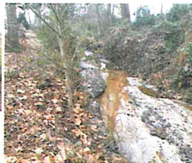
Phase I of the E. Grady Street City park stream restoration looking downstream.
