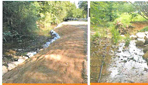
McLellan Creek Bank Stabilization and Green Infrastructure
