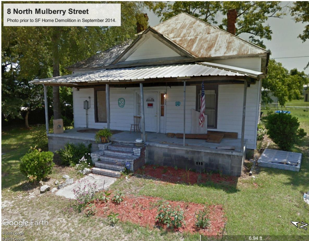
Picture 10: View of the subject site prior to the single family home demolition permitted under demolition permit #17. This single family residence was permitted for demolition on September 18, 2014.
