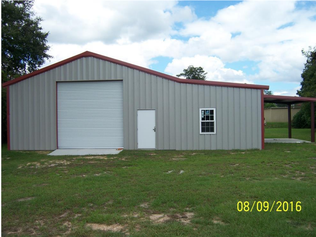
Picture 9: View of the subject site prior to the renovations permitted under building permit #02012 and #02009, previously a metal warehouse building with a one bedroom apartment.
