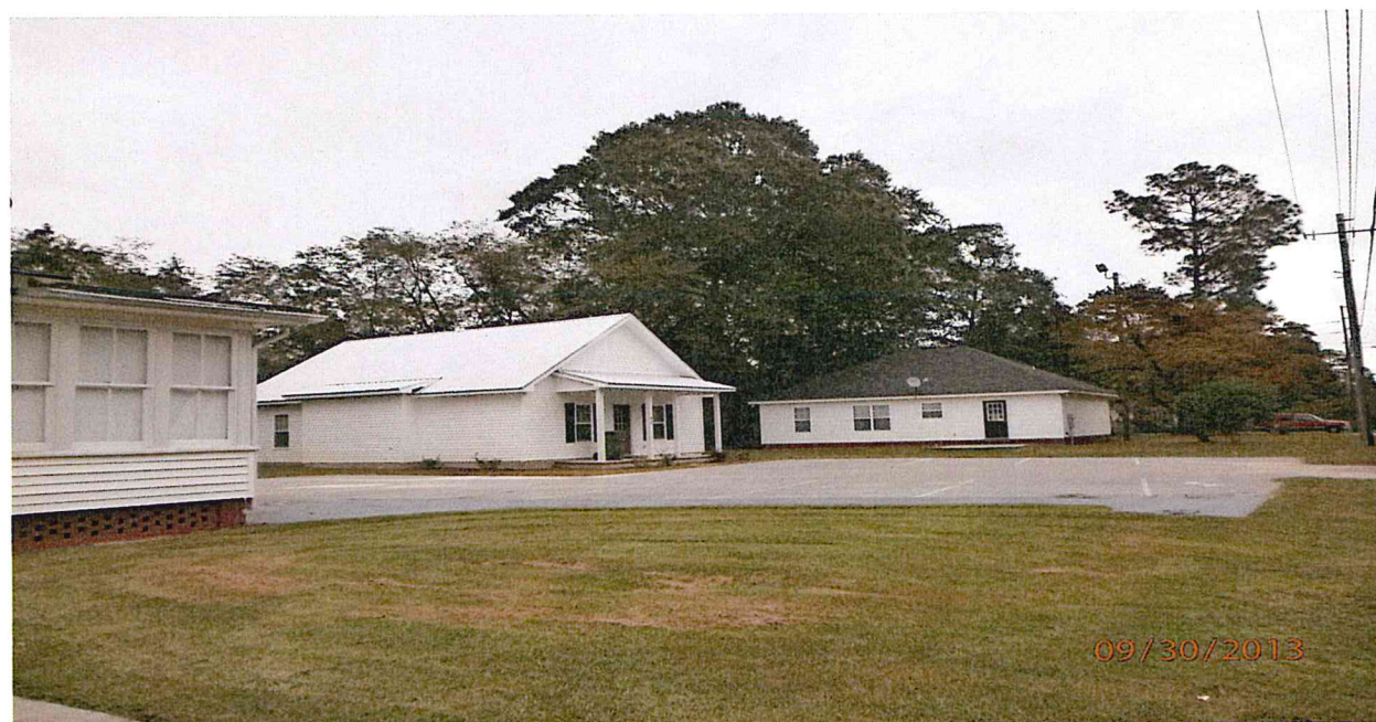
Storage building and apartment in rear of subject site
