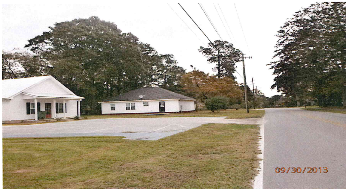
North view from side of subject site.
