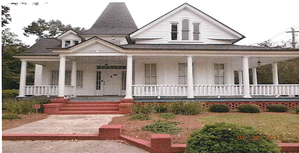
Front view of subject site from Zetterower Ave.
