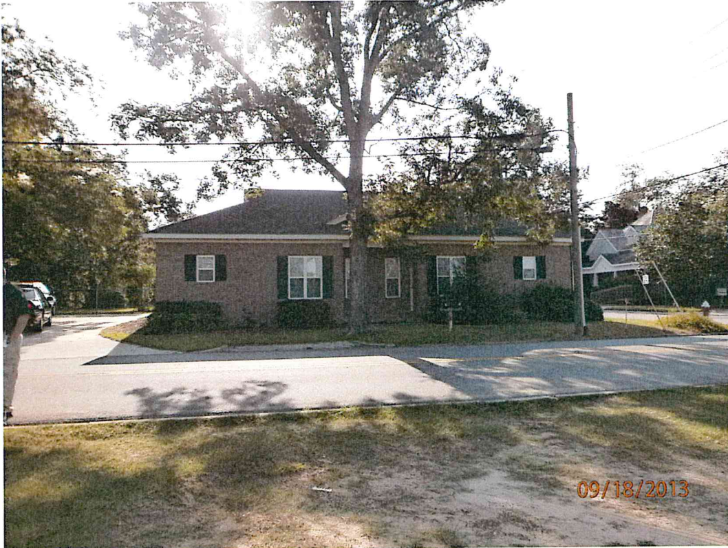
Figure 5: Eastern view from site fronting S. Mulberry Street.
