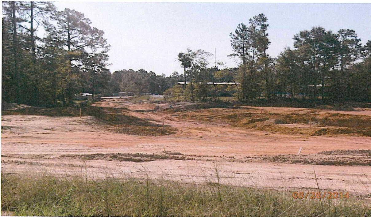
Figure 6: Access road being built from the subject site onto Highway 301 South.
