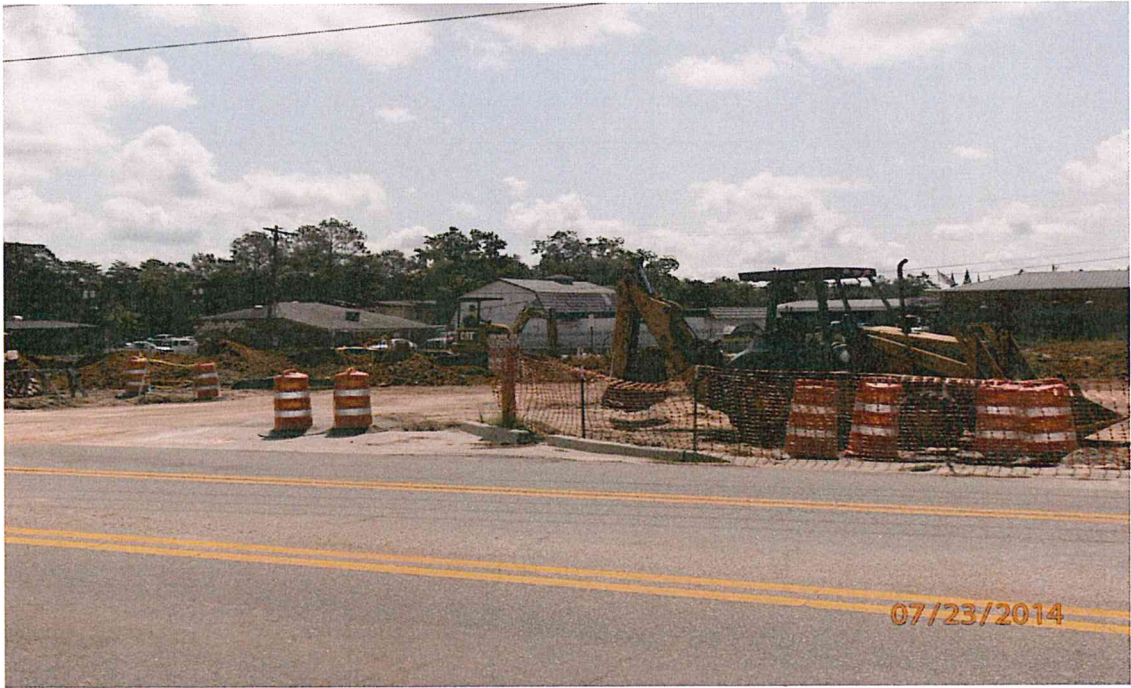
PHOTO 2: Existing Entrance on Chandler Road
