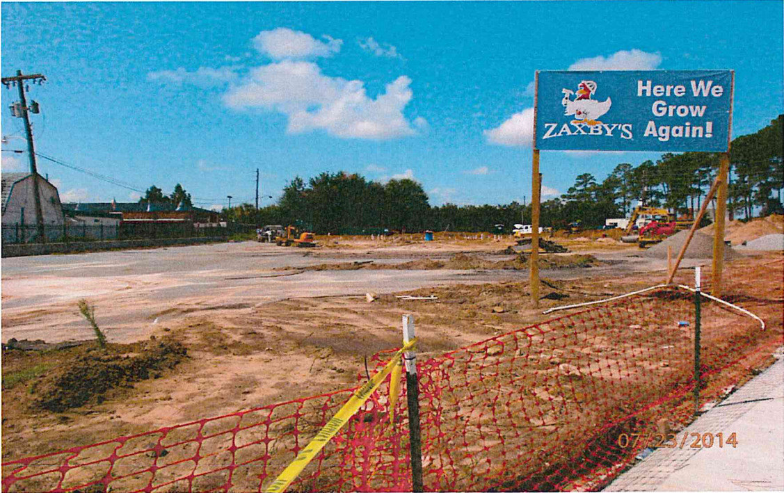
PHOTO 1: Subject Site from corner of Chandler Road and Georgia Ave.
