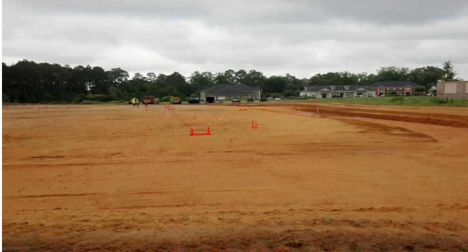
Figure 1: South Western View of Subject Site from Brampton Avenue.
