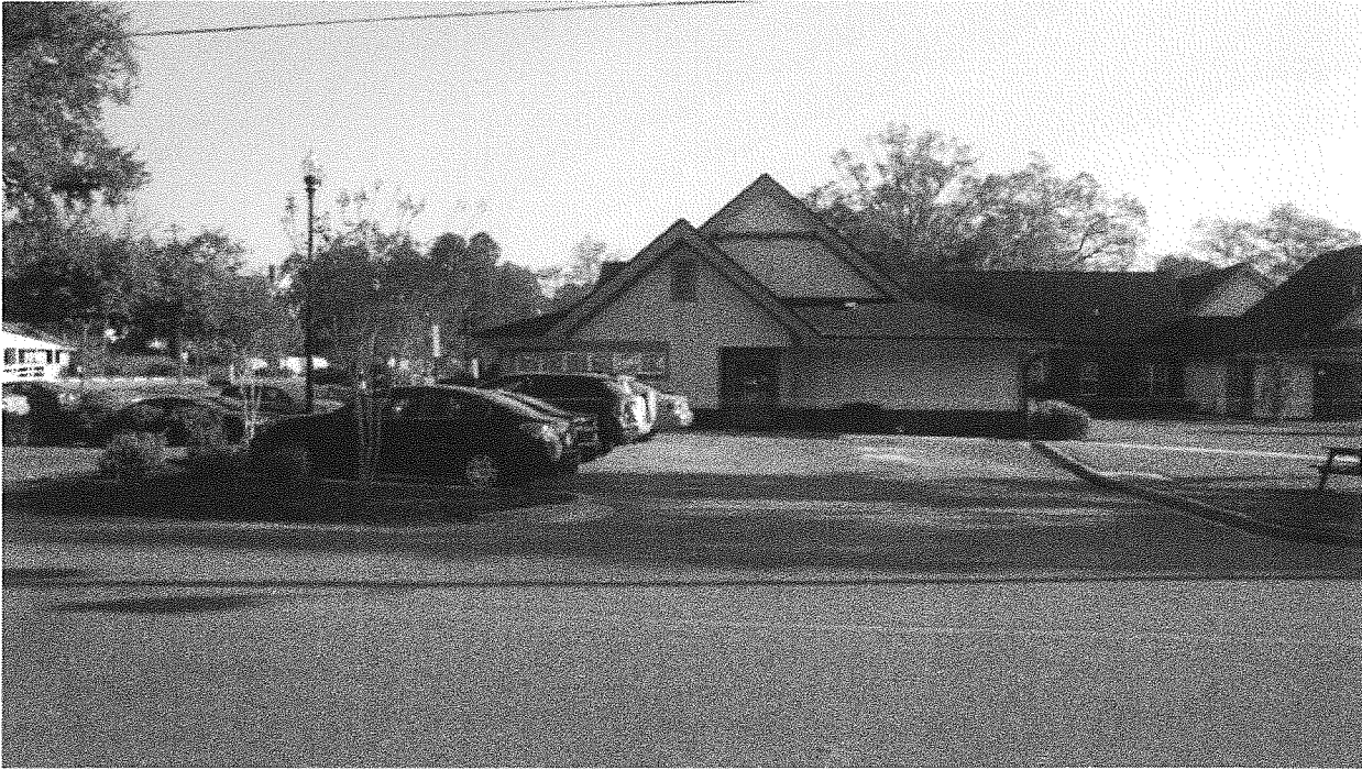
Figure 1b: Subject Property (Area of Proposed Expansion))
