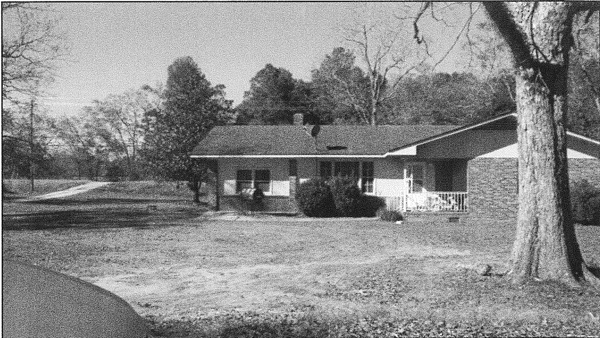
Figure 4: Adjacent property to the south that was recently annexed at R4.
