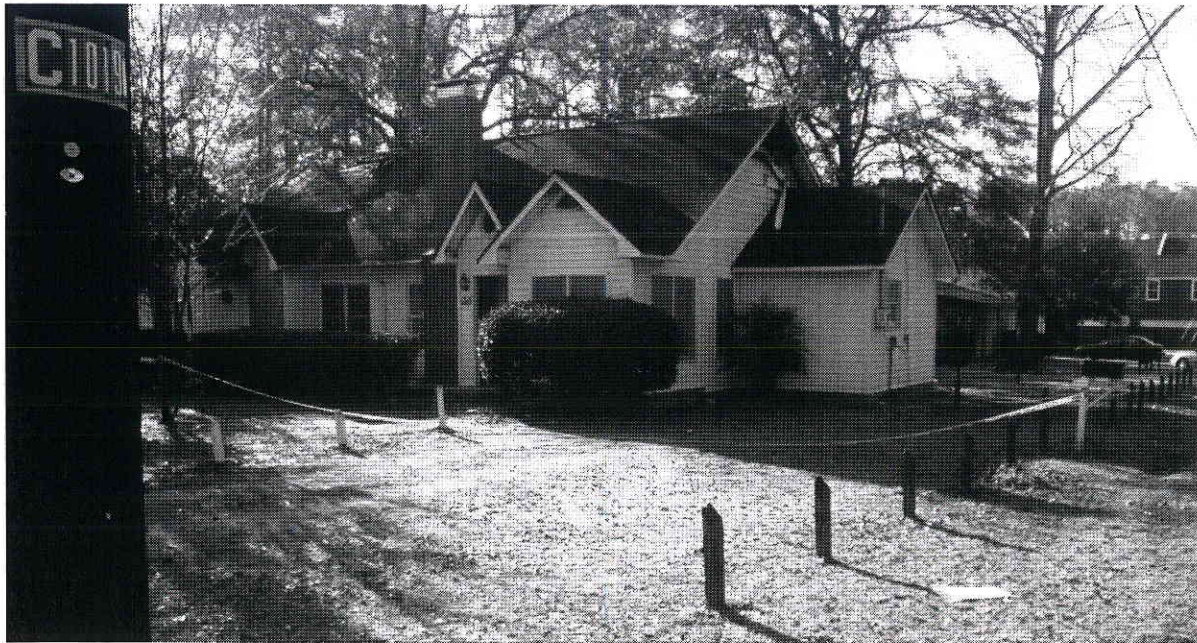
Figure 2b: Surrounding Land Uses: Abandon Duplex (north of subject parcel)
