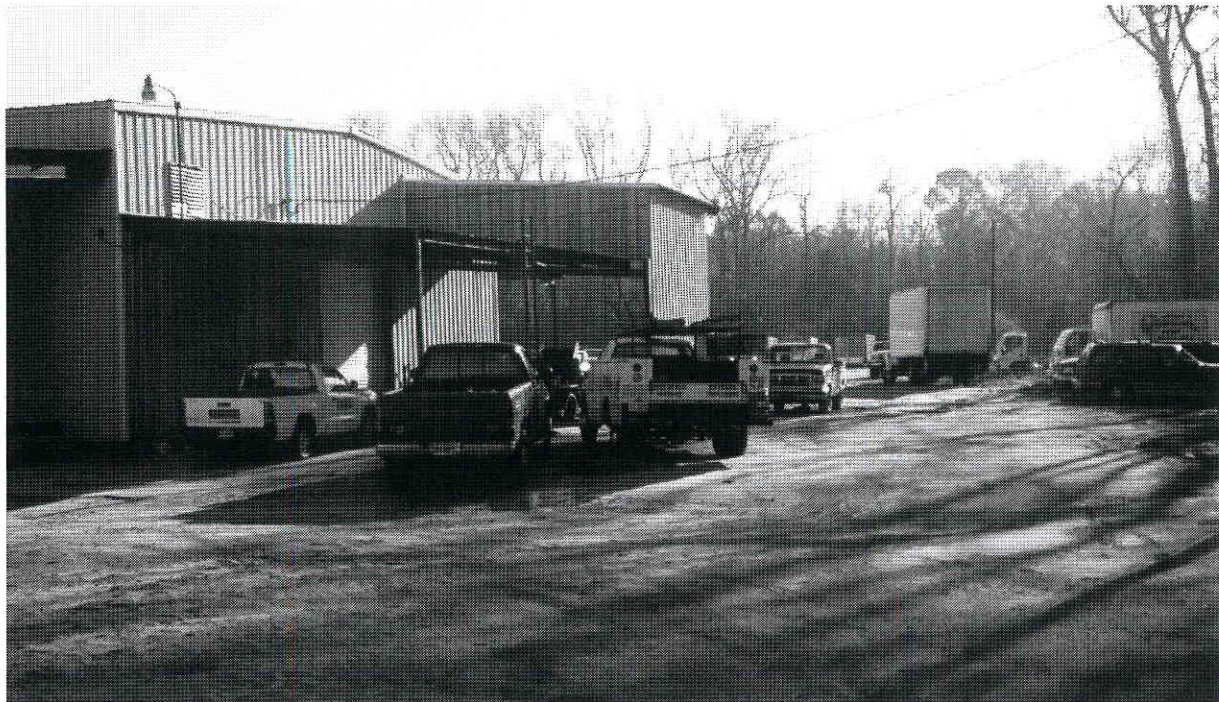
Figure 2b: Surrounding Land Use: B&S Steel (LI) located directly behind the subject parcel
