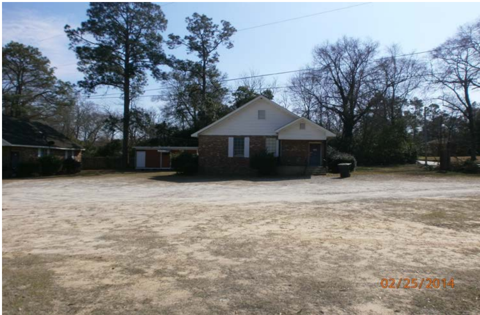
Figure 2: Southern view of Subject Property from northern side of Subject Property
