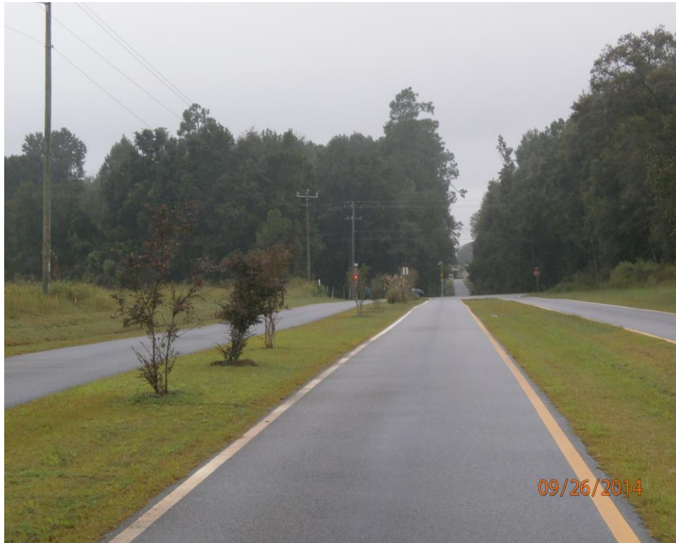
Photo 5: West view from S&S Railroad Bed Road with Subject Site to the North, Cawana Road and S&S Greenway Trail crossing to the West and undeveloped adjacent property to the South that was recently rezoned to R4 & R10.
