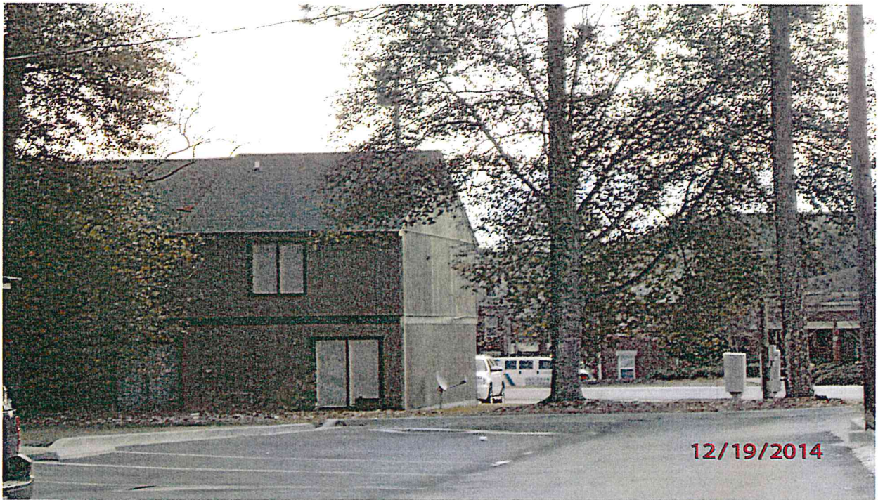
Photo 4: Student Housing to the South of Subject Site
