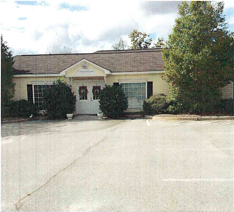
Picture 2 Rear of Subject Property Facing North
