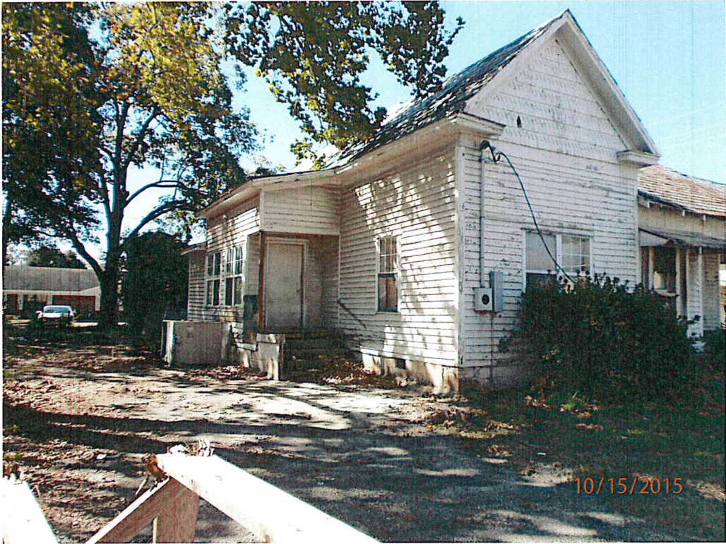
Picture 2 Back of Tax Parcel S19 000050 000 Facing West (Demolition Request)
