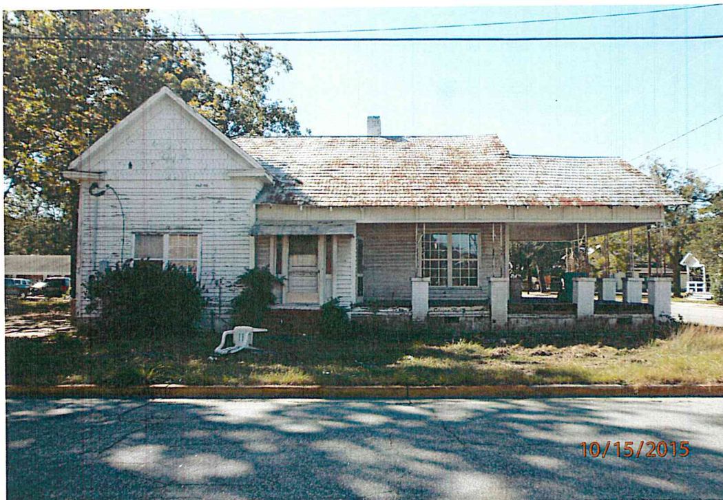
Picture 3 Side of Tax Parcel S19 000050 000 Facing West (Demolition Request)
