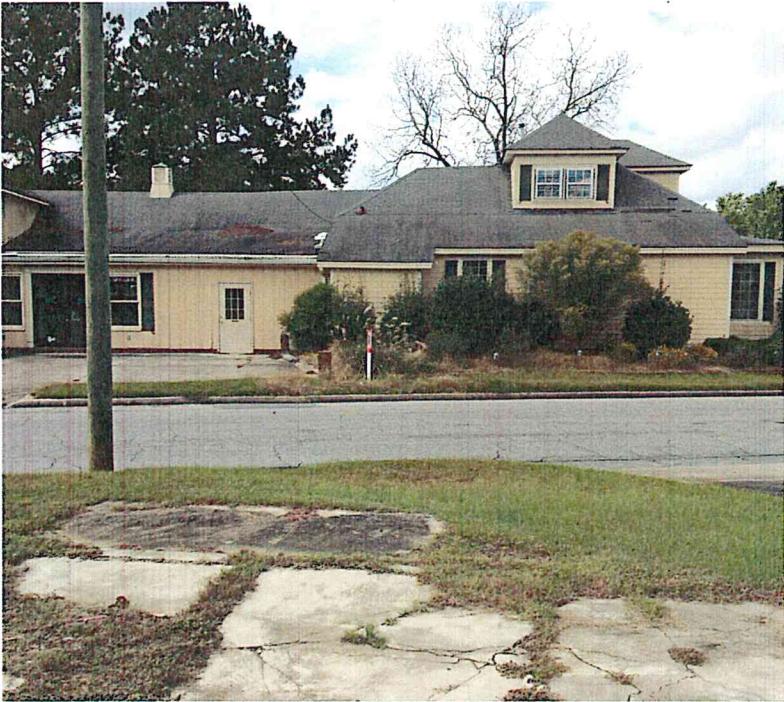
Picture 1 Subject Property Facing West
