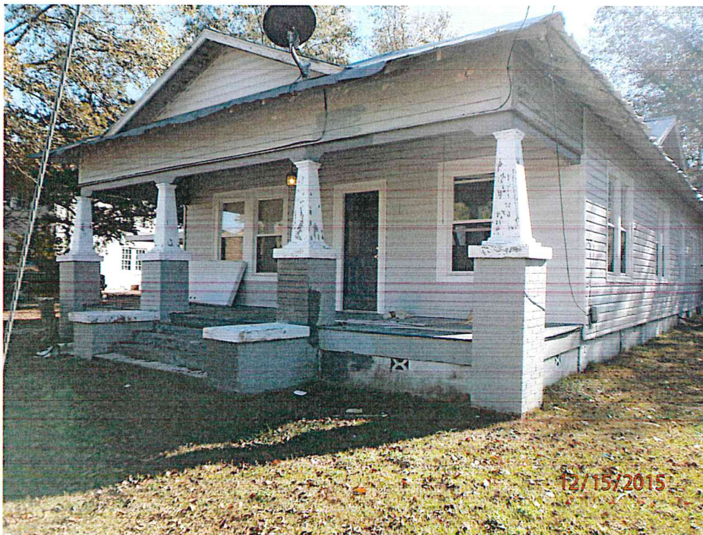
Picture 2 Tax Parcel S19 000030 000 Facing Southeast (3 bedrooms 2 bathrooms)
