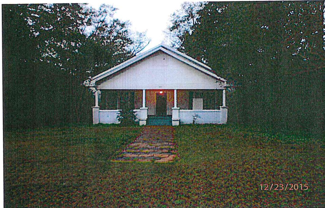
Figure 1: The Subject Property from Broad Street
