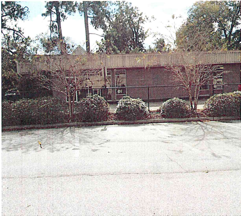
Picture 6 Adjacent Property Facing South
