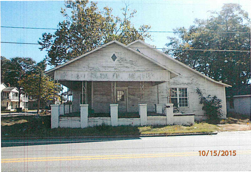
Picture 1 Tax Parcel S19 000050 000 Facing East (Demolition Request)
