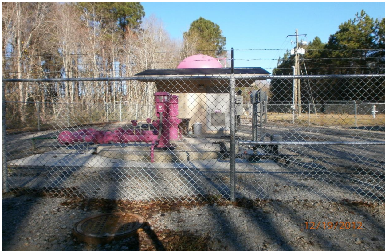
Figure 3: City of Statesboro Lift Station with Purple Pipes.
